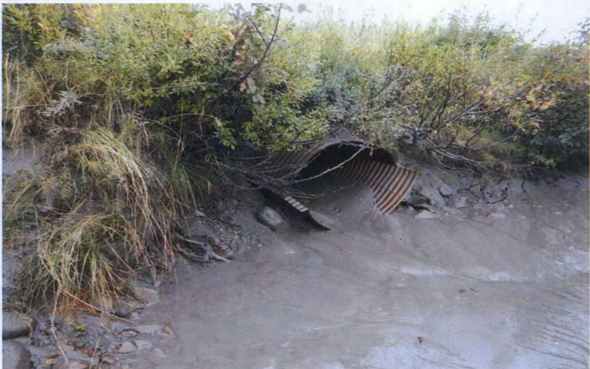
Figure 7. FPC 1, 48-inch culvert, culvert outlet view.
