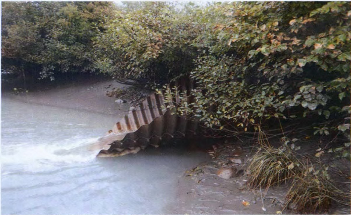
Figure 6. FPC 1, 72-inch culvert, culvert outlet view.
