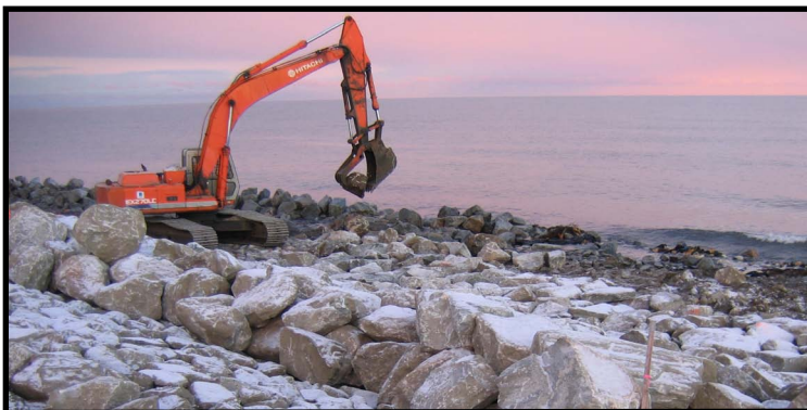
A contractor places rock revetment to protect Shishmaref from coastal erosion.
