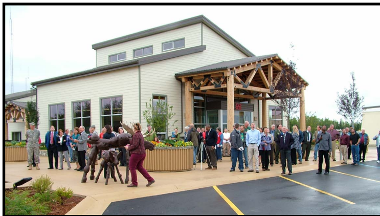
The Chena River Lakes Flood Control Project office, renovated with $5.47 million in American Recovery and Reinvestment Act funds, used local contractors, craftsmen and materials.
