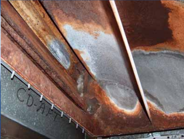
Rusted structural steel
