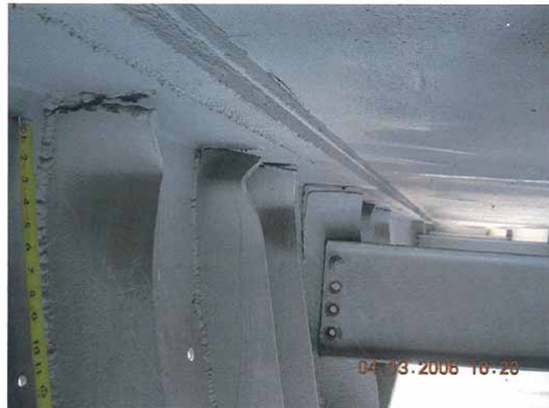
Bridge No. 0976 Structure Hillcrest Overcrossing Date 04/13/2006 Roll/Disk I Inspector Scarborough / Banse Frame 10 Buckled Stiffeners on Left Exterior Girder.
