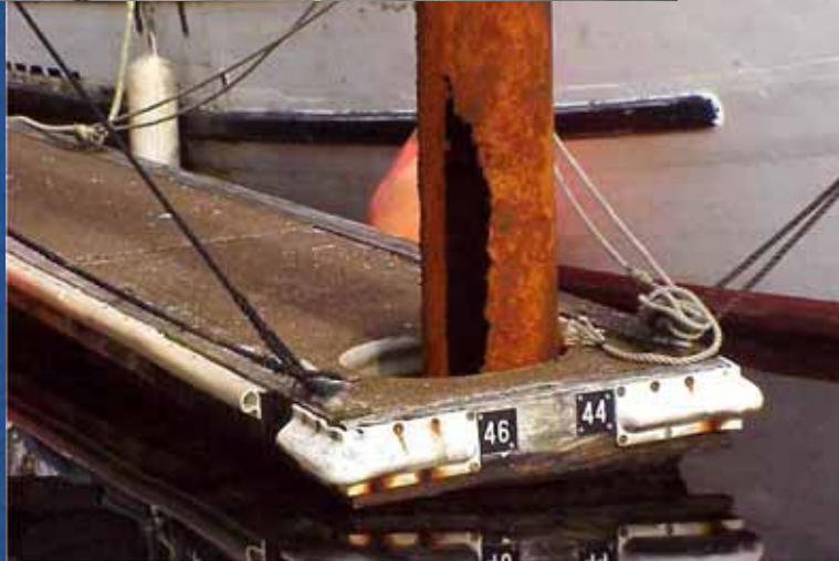
Corroded pile At Ketchikan
