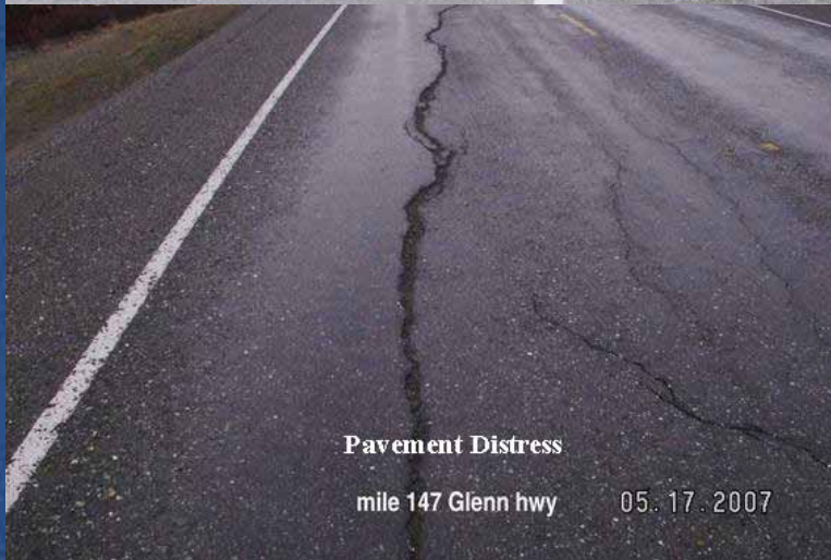
Typical Settlement Problem Common Throughout the Northern Region
