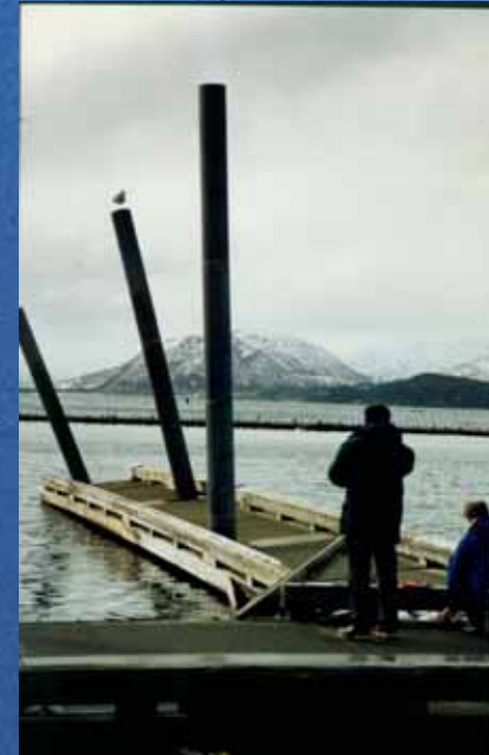
Bent piles at Kodiak
