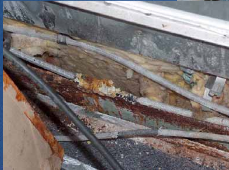
Corroded power cables
