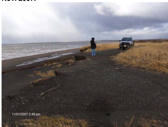
Photo 3: Roads in the old Port Heiden town site area continue to be cut off by erosion, Nov. 2007.
