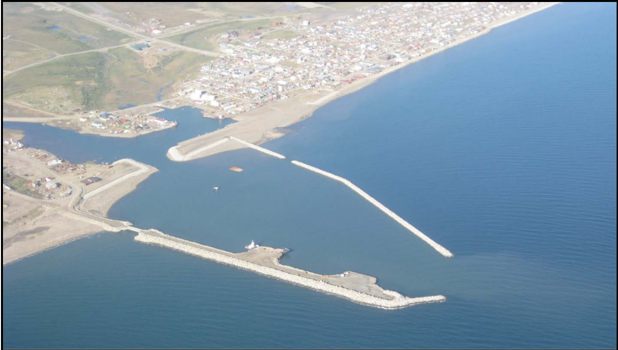
Figure 3. Aerial oblique view of current harbor configuration; view is towards the east-northeast.
