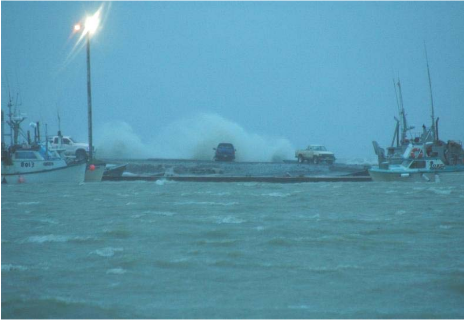
Photo 1. Storm waves breaking over the outer banks of the harbor.
