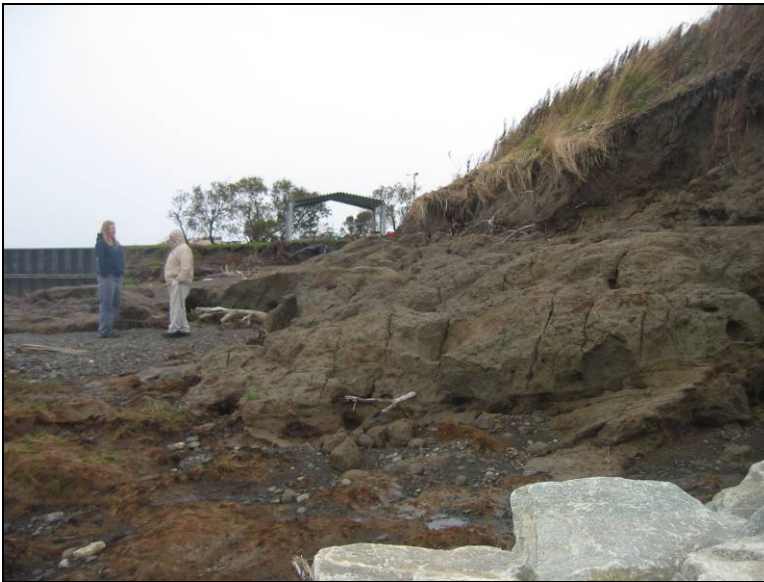
Photo 8. Erosion at the containment berm.
