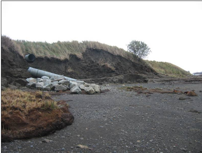
Photo 6. Containment berm 5 Sept. 2005.
