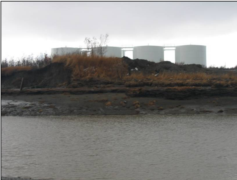
Photo 7. Bristol Alliance Fuel facilities as seen behind the eroding bank.
