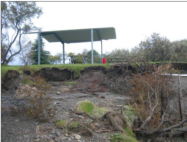
Photo 5. City Dock Side erosion at the park.
