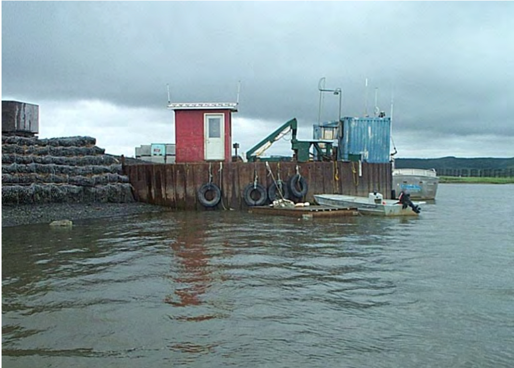
Loading dock adjacent to the fish processing plant.
