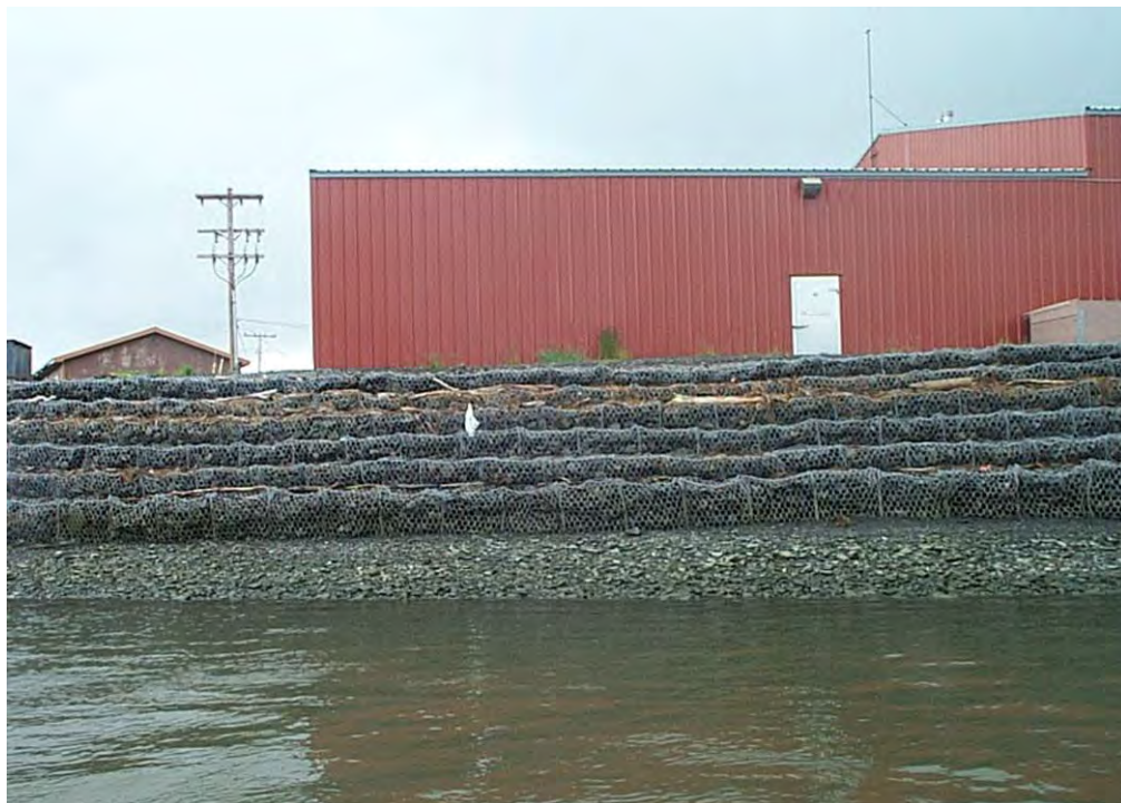
Existing gabion structure near the fish processing plant.
