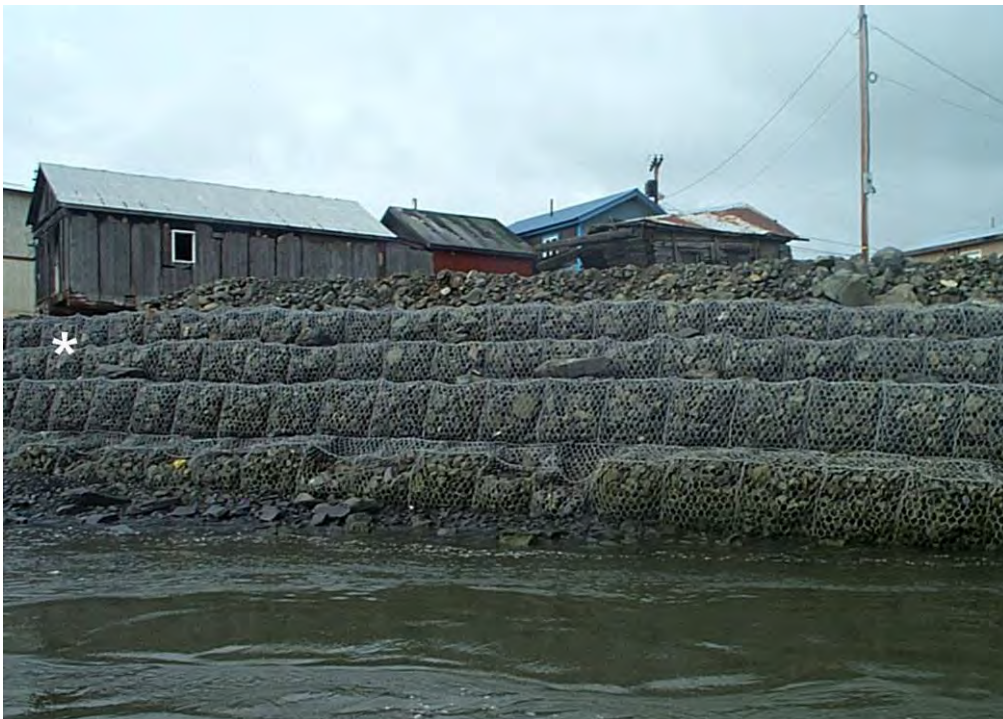
Structures threatened by coastal erosion. Note the extensive erosion near the structure in the left of the photograph (denoted by white star).
