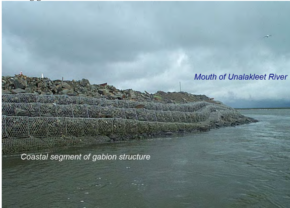
Coastal segment of existing gabion structure.
