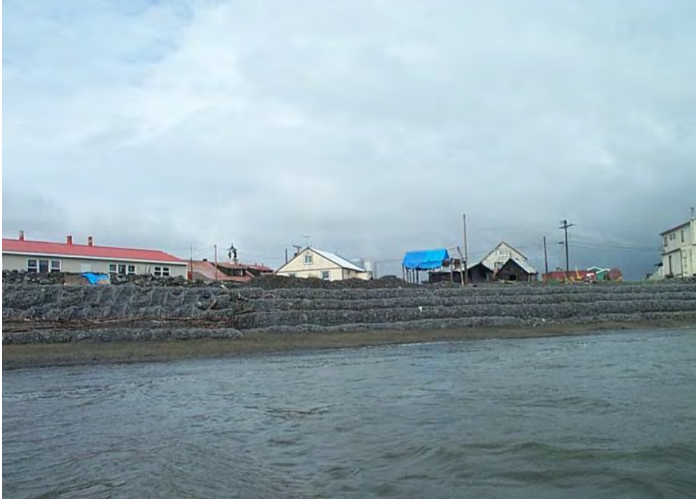
Structures threatened by coastal erosion.
