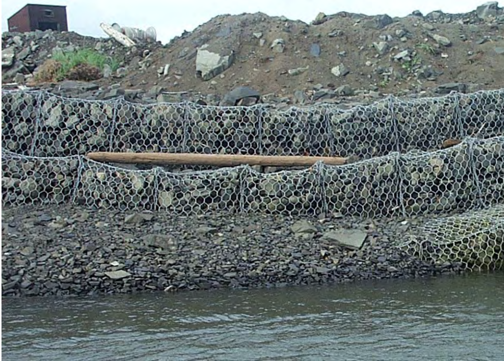
Existing gabion structure.
