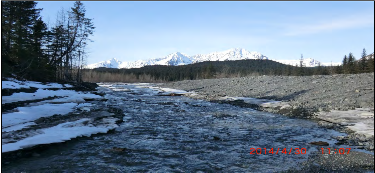
Figure 5: Looking northwest at the existing berm from the creek bed. Photo taken on 30 April 2014.
