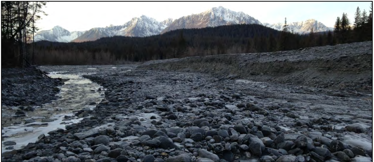
Figure 6: Looking northwest at the existing berm from the creek bed. Photo taken on 29 October 2014.
