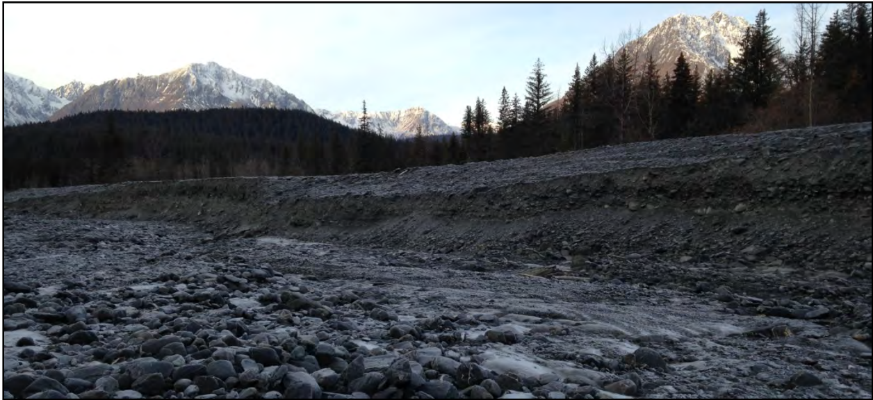
Figure 1: Looking northwest at the existing berm from the creek bed.
