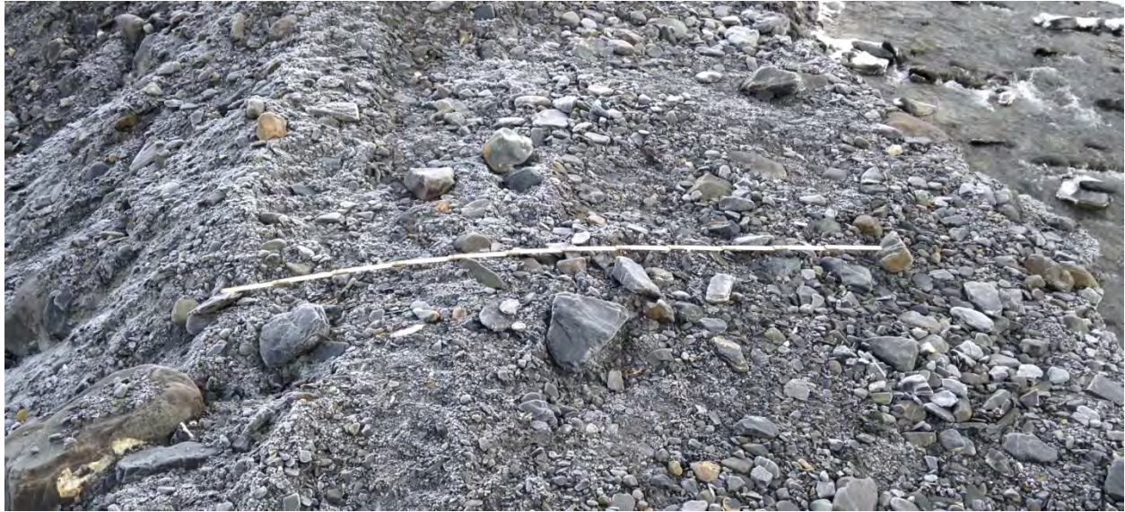
Figure 7. Eight-foot minimum crest width where erosion is most severe.
