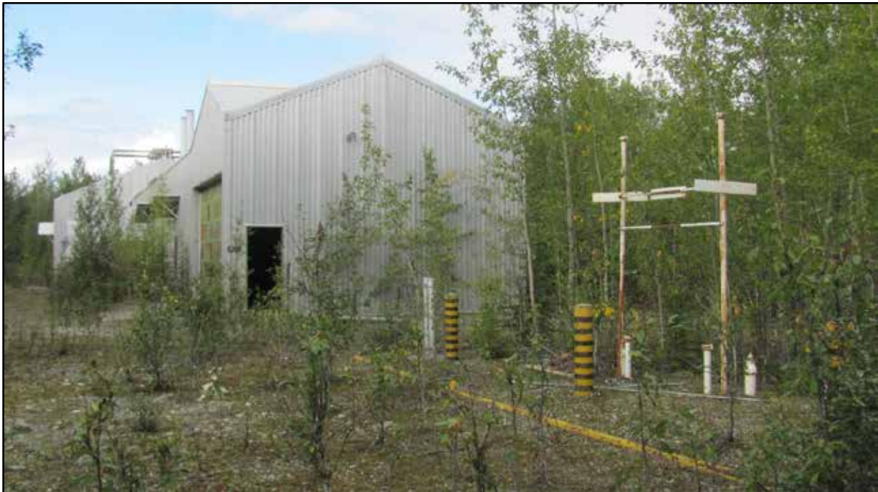
Timber Pump Station, 2015
