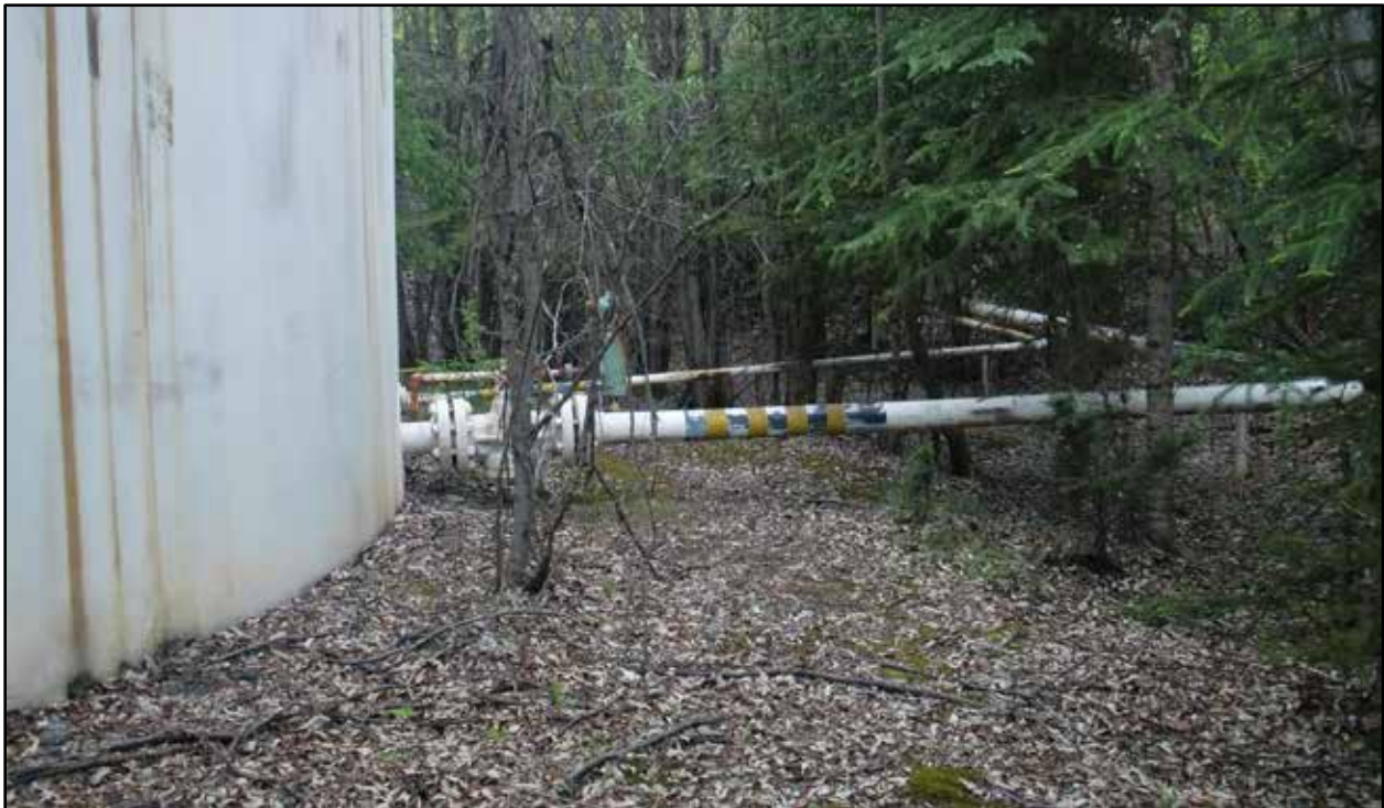
Figure 5. Timber Pump Station: Partial view of the 59,000-gallon AST with pipes and valves (May 2016).
