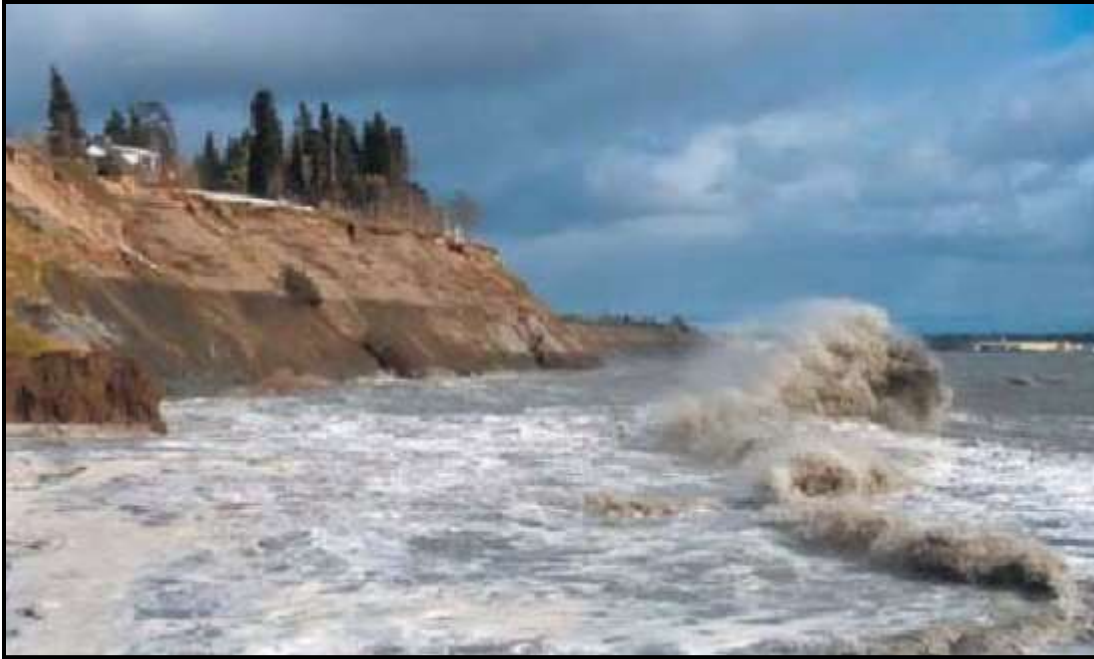
Figure 12. Waves during a Storm Event at Kenai Bluffs
