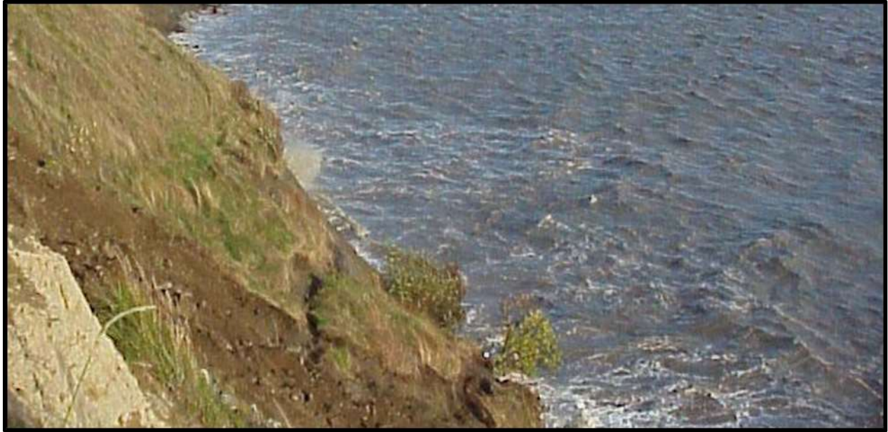
Figure 9. Kenai River estuary at the base of the eroding bluff showing highly turbid water.
