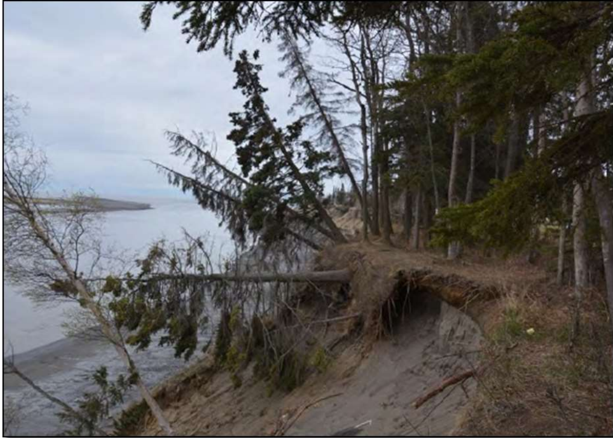
Figure 13. Trees and Root Balls Failing
