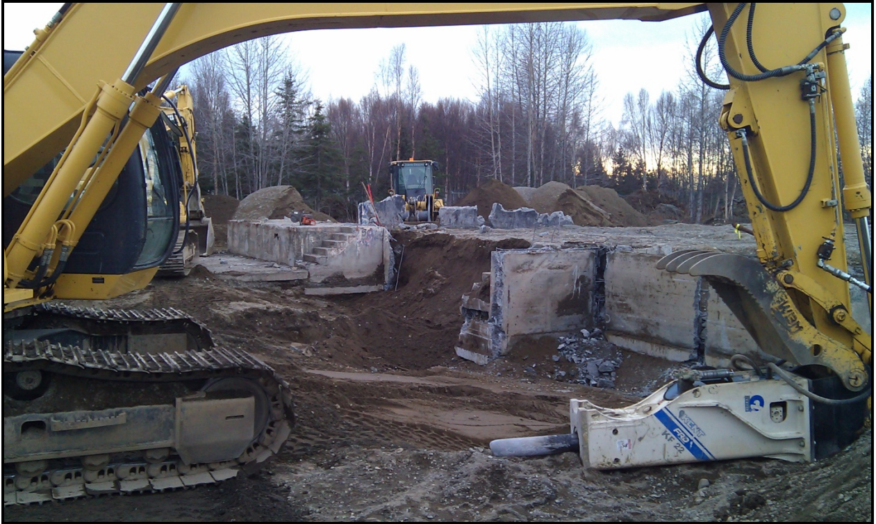
Figure 3. Demolition of a concrete structure at the Wildwood AFS.
