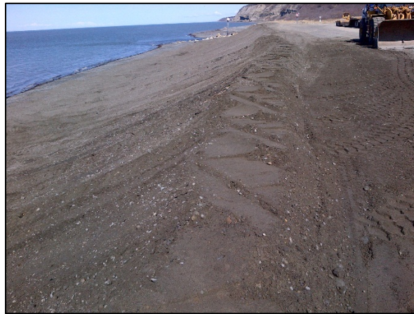
Photograph 6. Dredged material contoured to match the existing shoreline and beach contours
