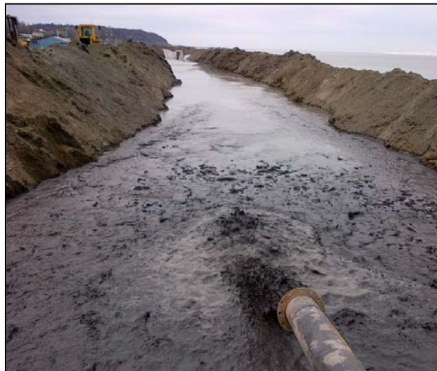
Photograph 4. Dredged material from the mooring basin being discharged into the dewatering basin
