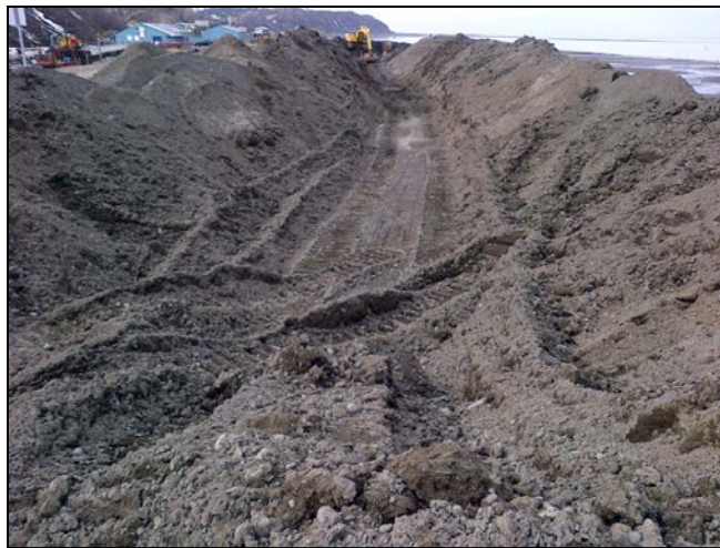
Photograph 2. Constructing the dewatering basin, Ninilchik SBH
