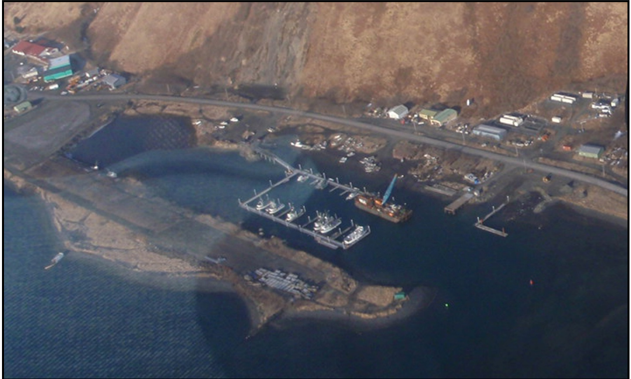
Figure 2-1. A 2010 aerial view of the Old Harbor small boat harbor.
