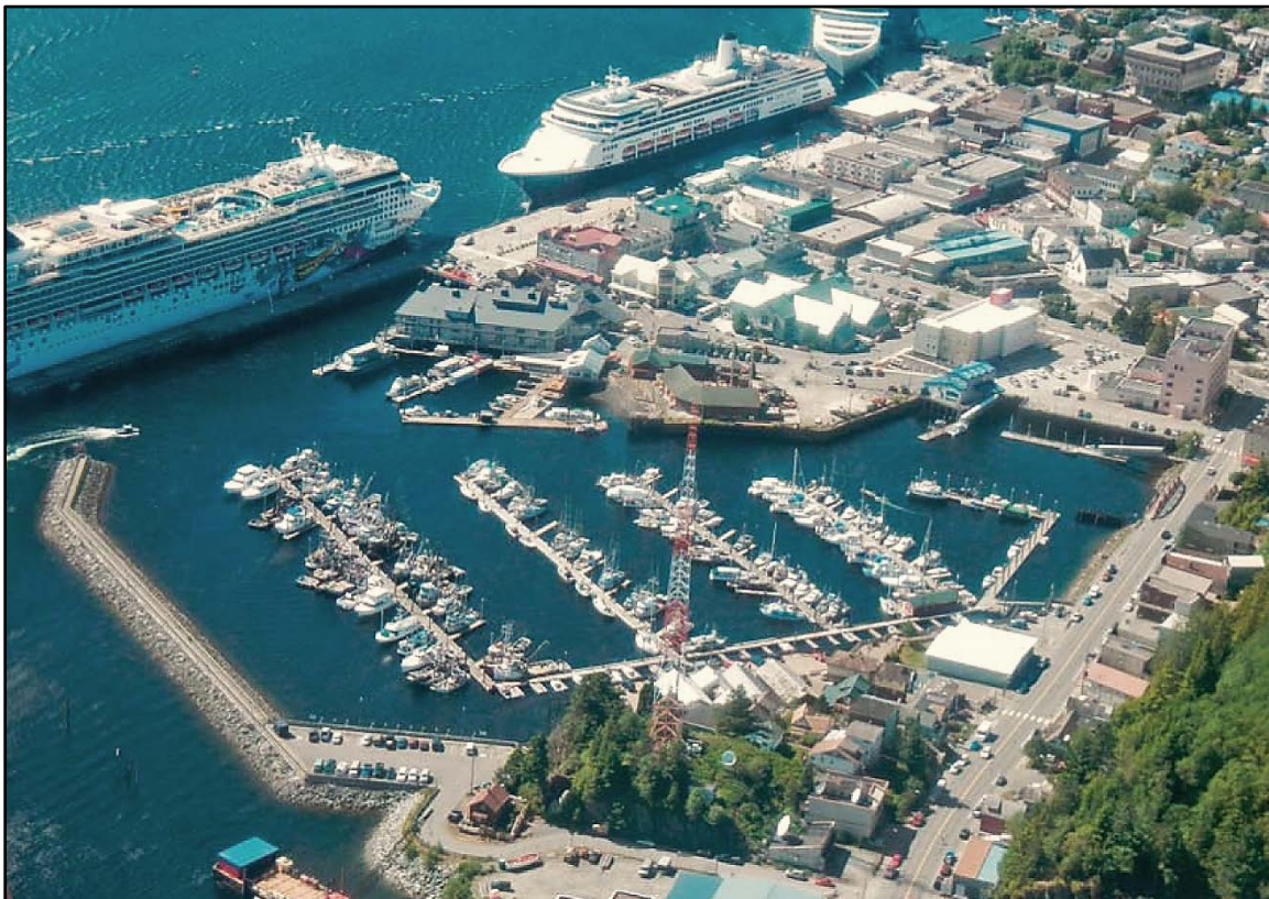
Figure 6. An aerial view of Thomas Basin harbor from the southeast, showing the dense urban development surrounding the harbor (undated).
