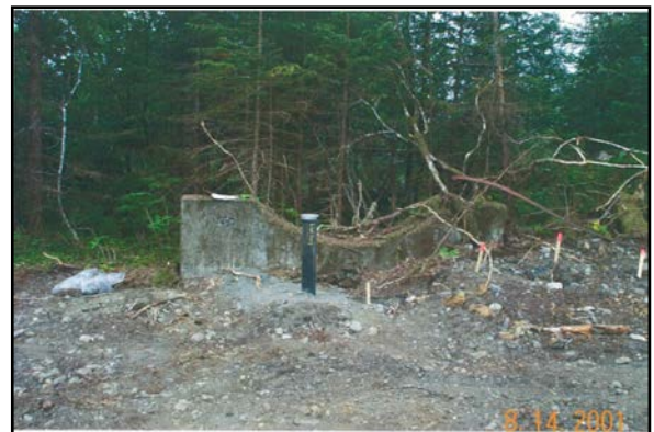
L3 - Typical AST Tank Foundation (ENSR 2003b)
