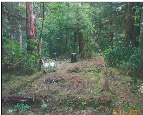
C7 - Concrete Powerhouse Foundation (ENSR 2003b)
