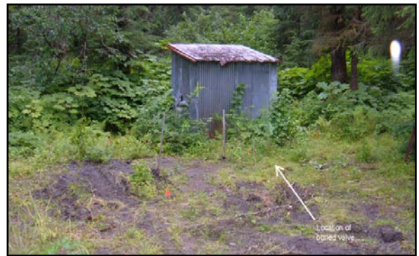
L2 - Separator Tank (USACE 2006)
