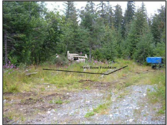
L5 - Pump House Foundation (USACE 2006)
