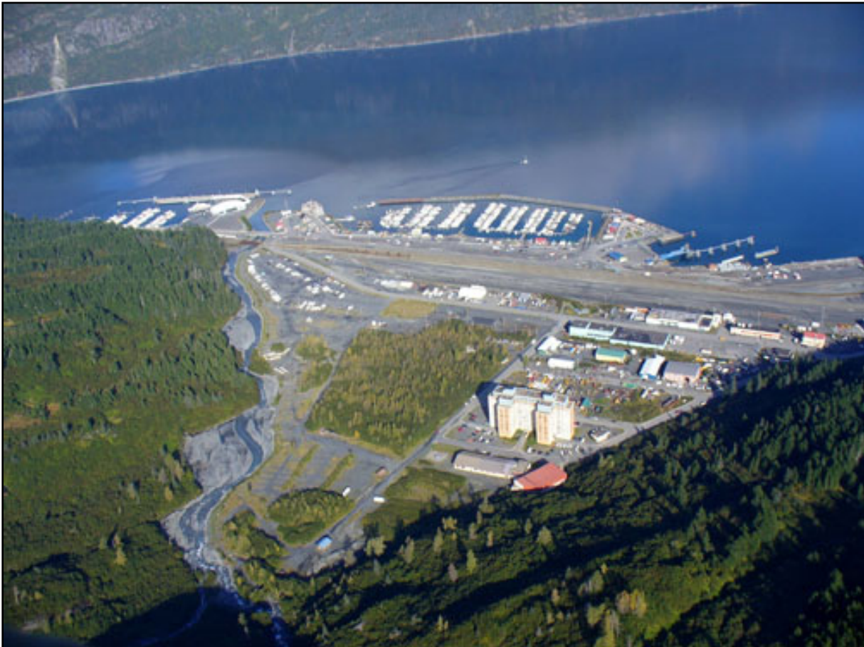
Figure C-7. Whittier Marine Facilities
