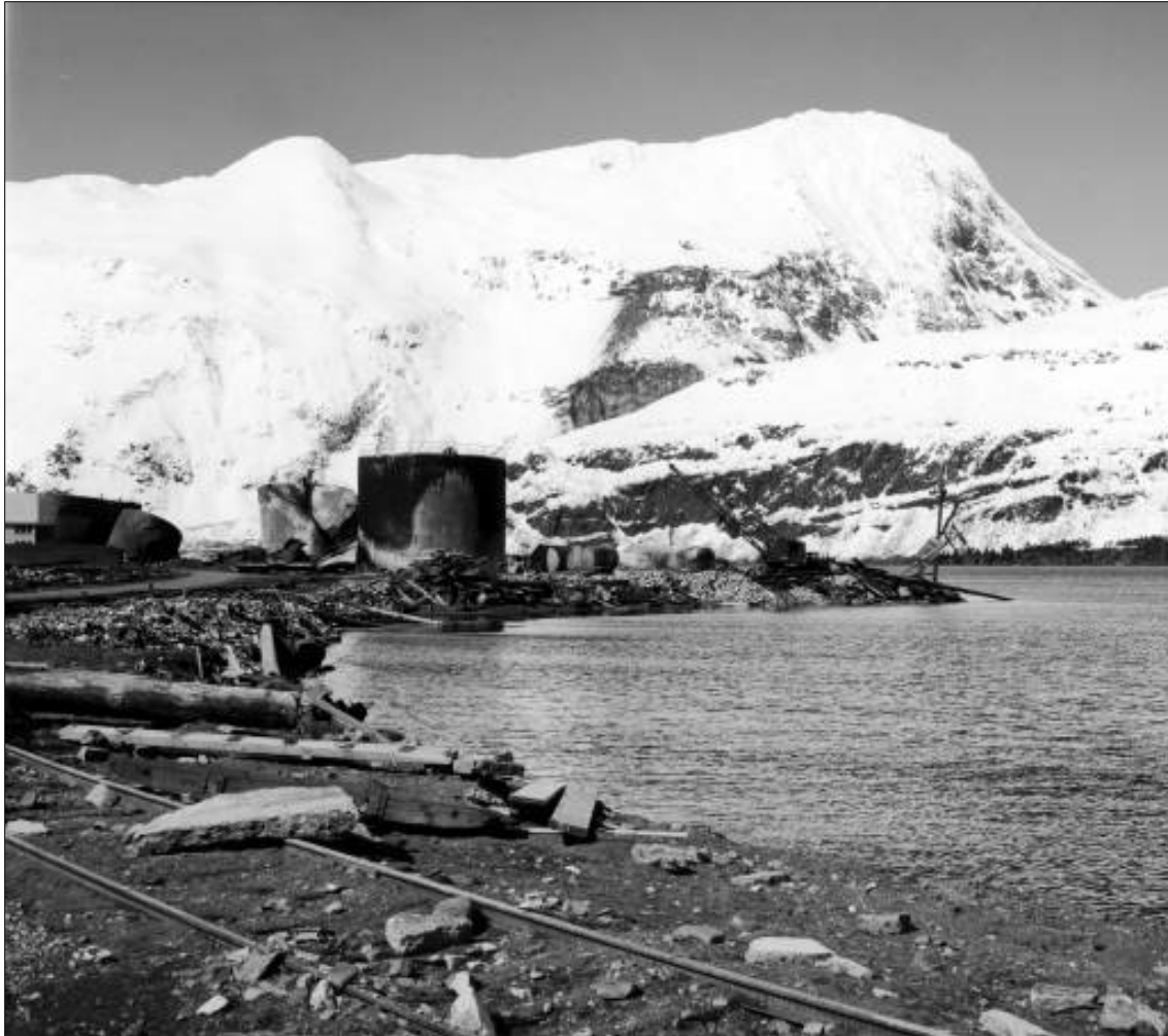
Figure E-1: March 27, 1964, Photo Showing Damage to Fuel Tanks After Earthquake [photo appears to be facing northwest into the head of passage canal (ADA 2018).]
