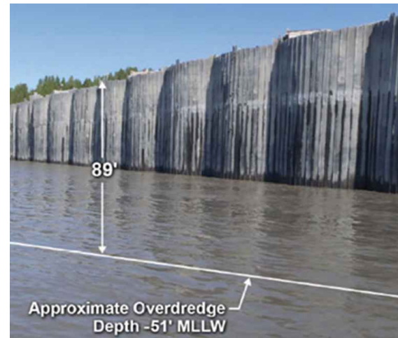
WATERSIDE VIEW OF THE NORTH EXTENSION OCSP CONTAINMENT WITH ORIGINAL DESIGN MUDLINE DEPTH
