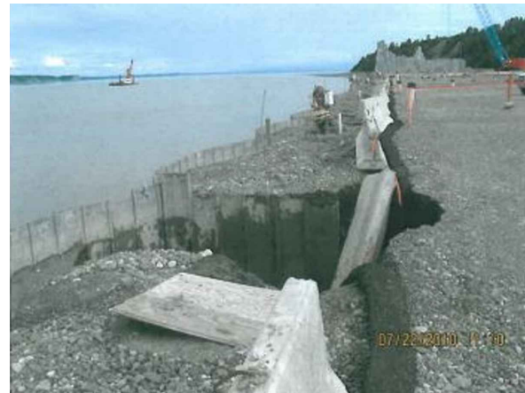
SUBSIDENCE OF IMPOUNDED MATERIALS AT THE FACE WALL OF OCSP CELL 66 ILLUSTRATING MATERIAL LOSSES THROUGH THE FACE SHEET INTERLOCKS (ICRC 2010)
