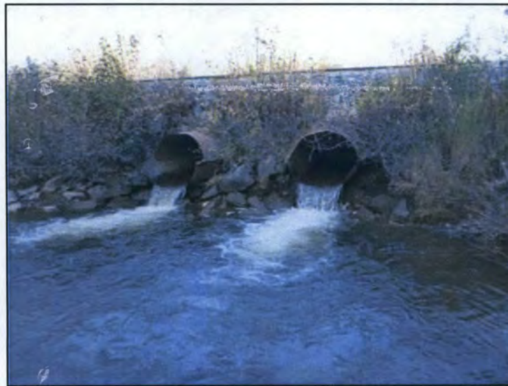
Inset 2. Perched 48-inch culverts on Explorer Creek, outlet view. October 3, 2016.
