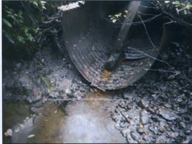
Inset 6. Poor quality culvert on unnamed tributary to Placer River. September 6, 2016.
