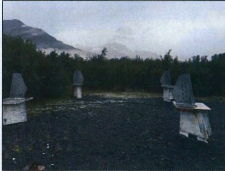
Inset 1. Abandoned microwave tower pad. September 6, 2016.
