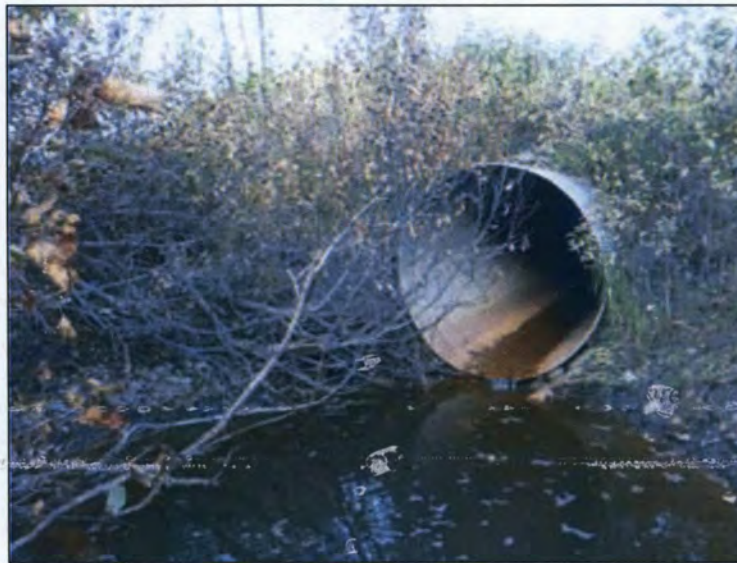
Inset 4. Perched culvert on unnamed tributary to Placer River. September 6, 2016.
