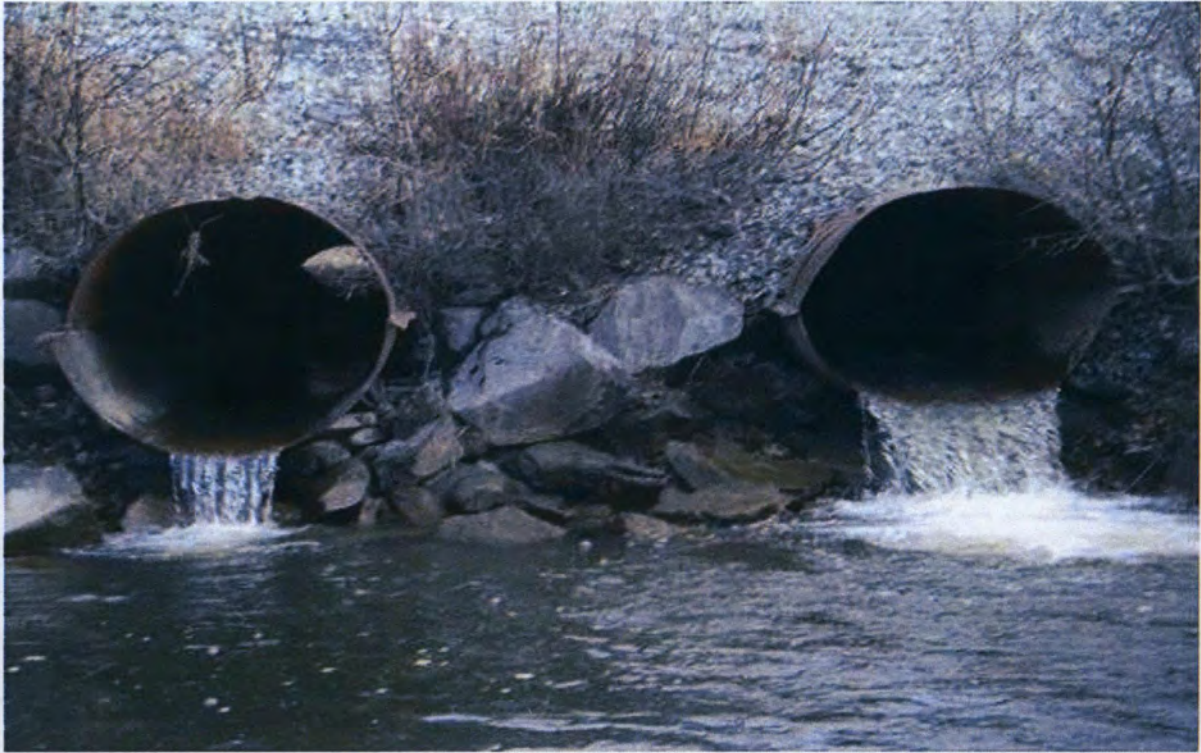
Figure 4. FPC 3, Explorer Creek culverts, outlet view. Photograph taken October 2008.
