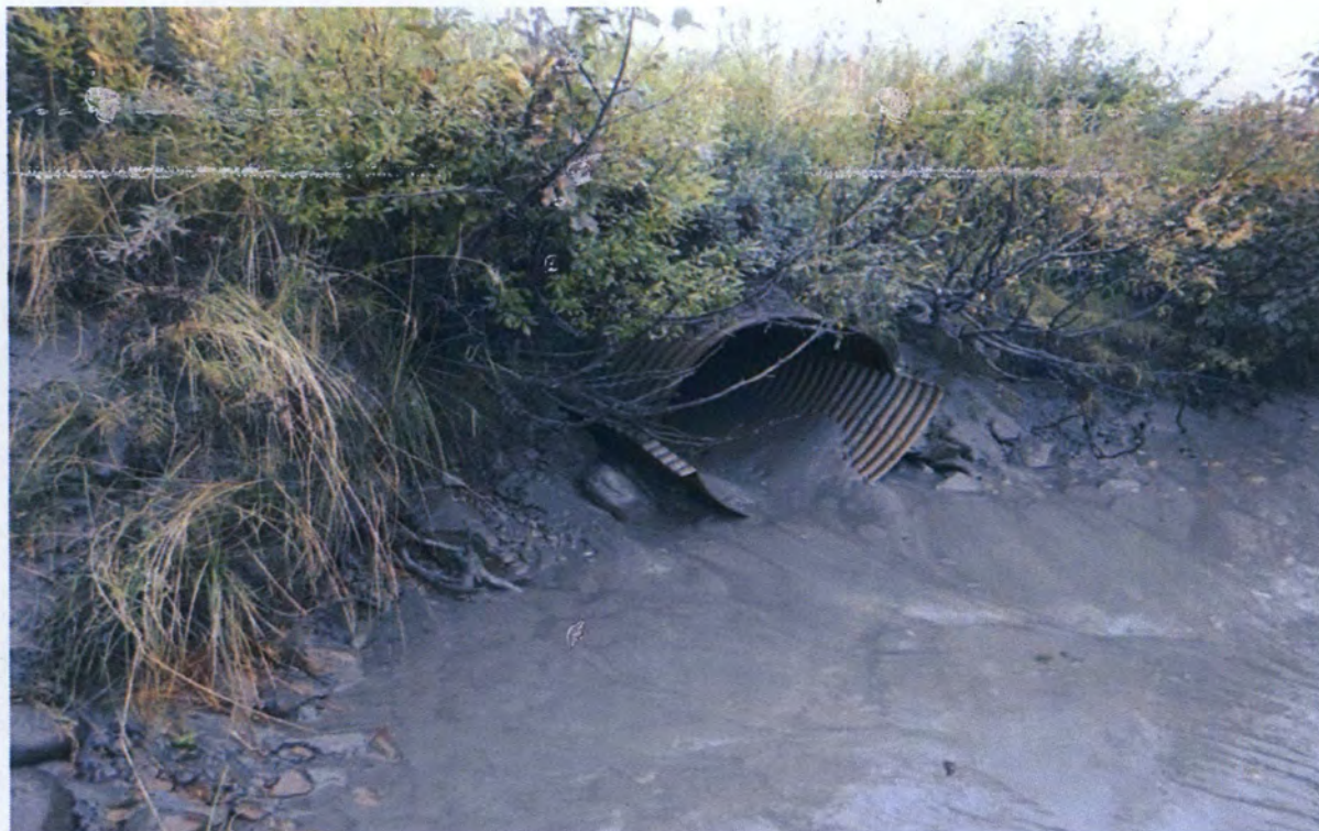
Figure 7. FPC 1, 48-inch culvert, culvert outlet view.
