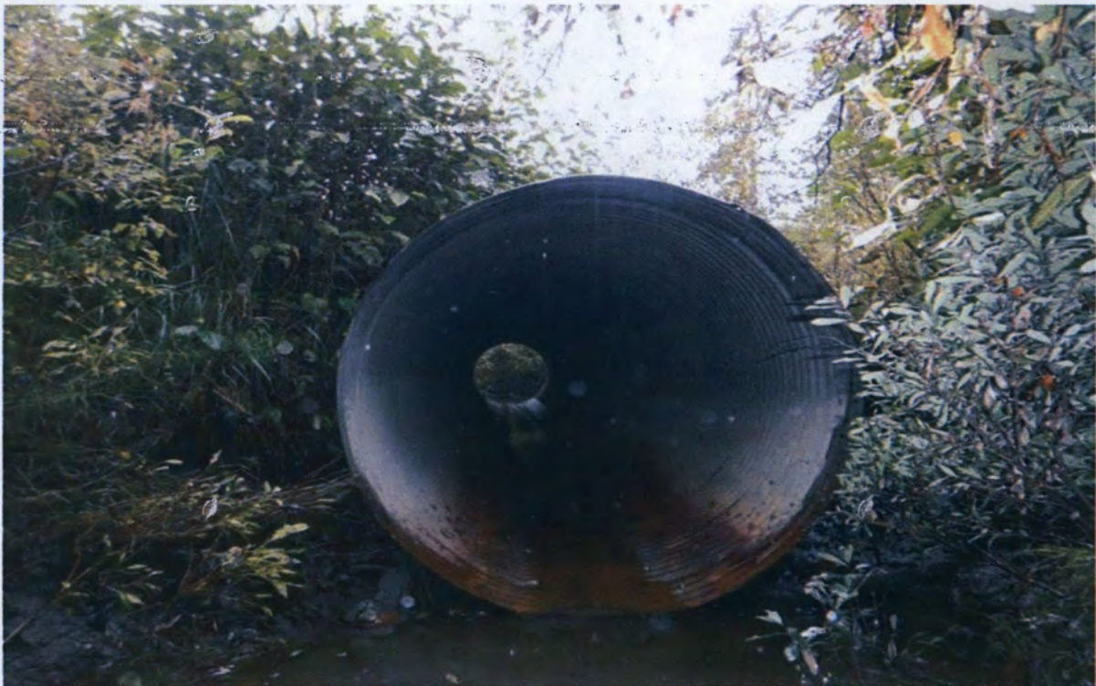
Figure 5. FPC 2, culvert inlet view.
