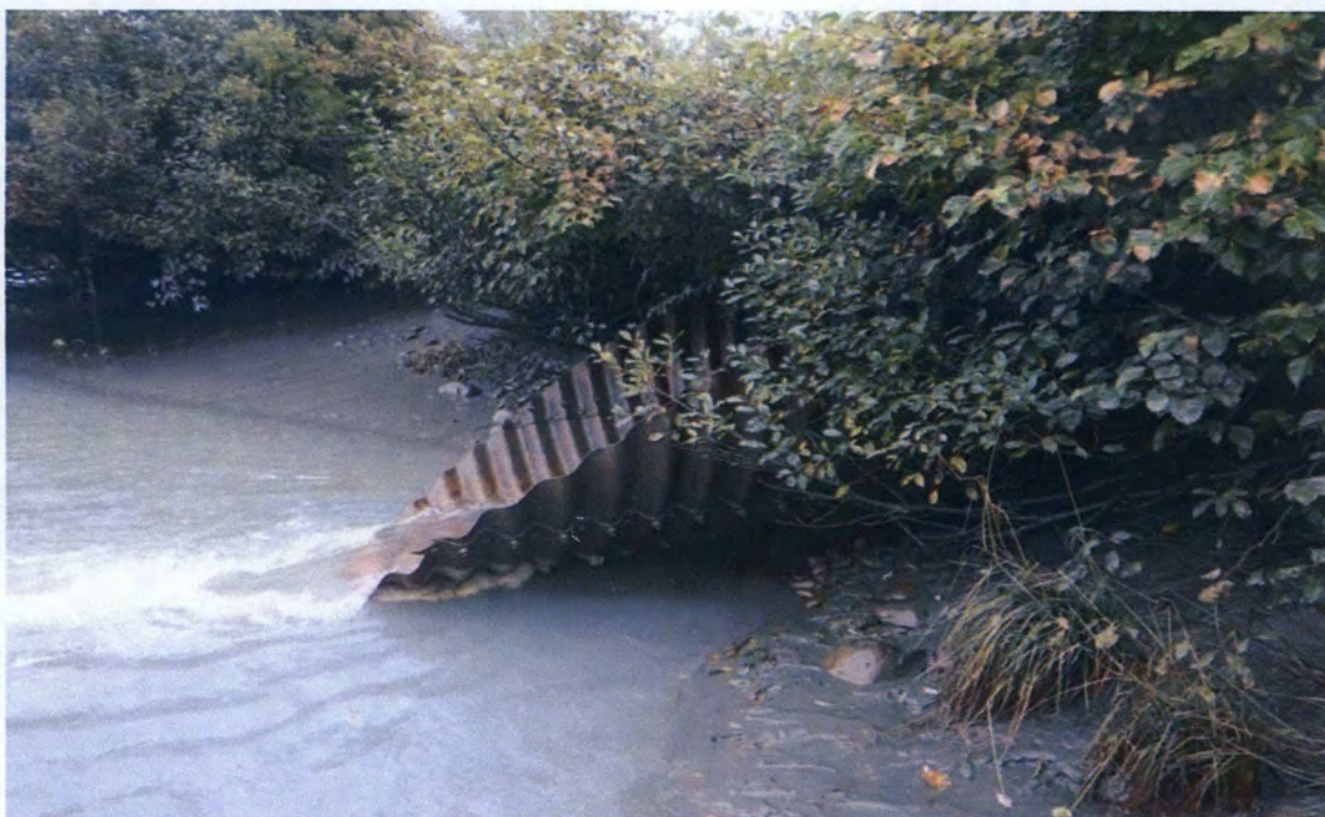
Figure 6. FPC 1, 72-inch culvert, culvert outlet view.
