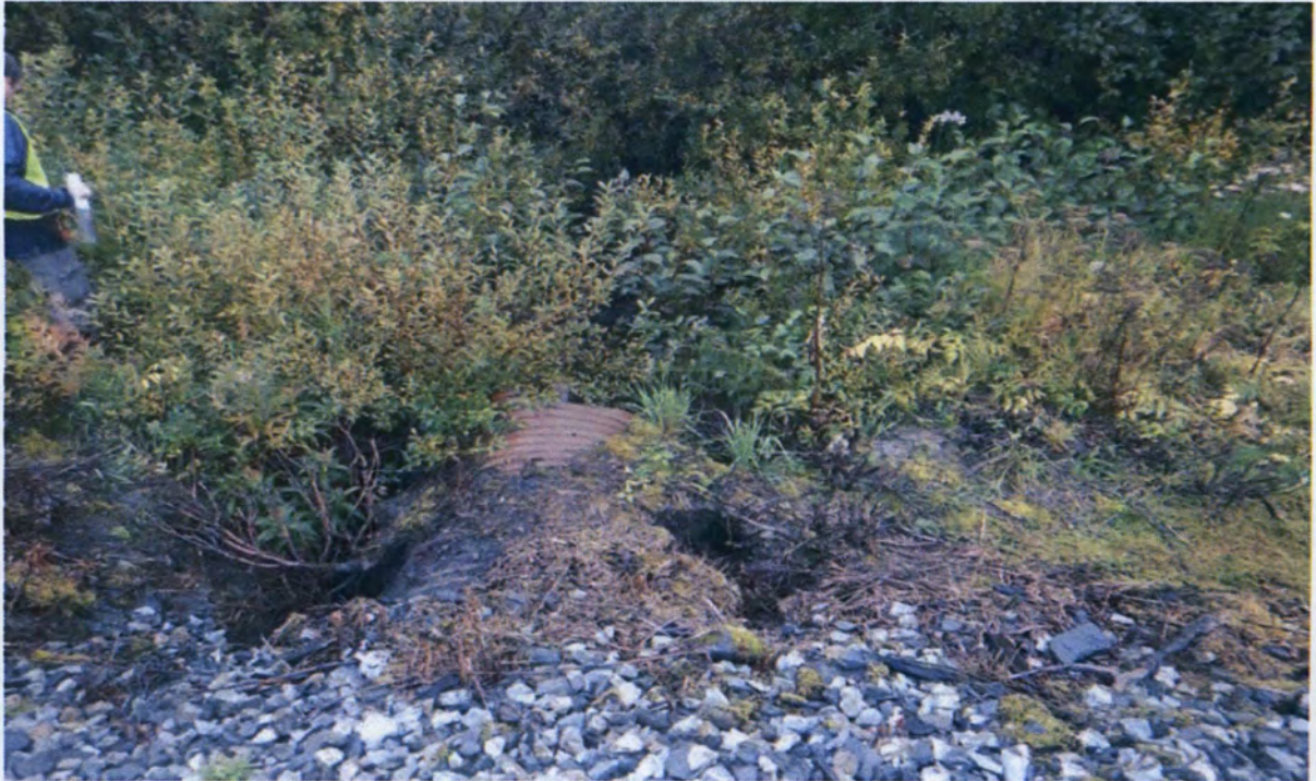
Figure 8. FPC 4, culvert outlet view.
