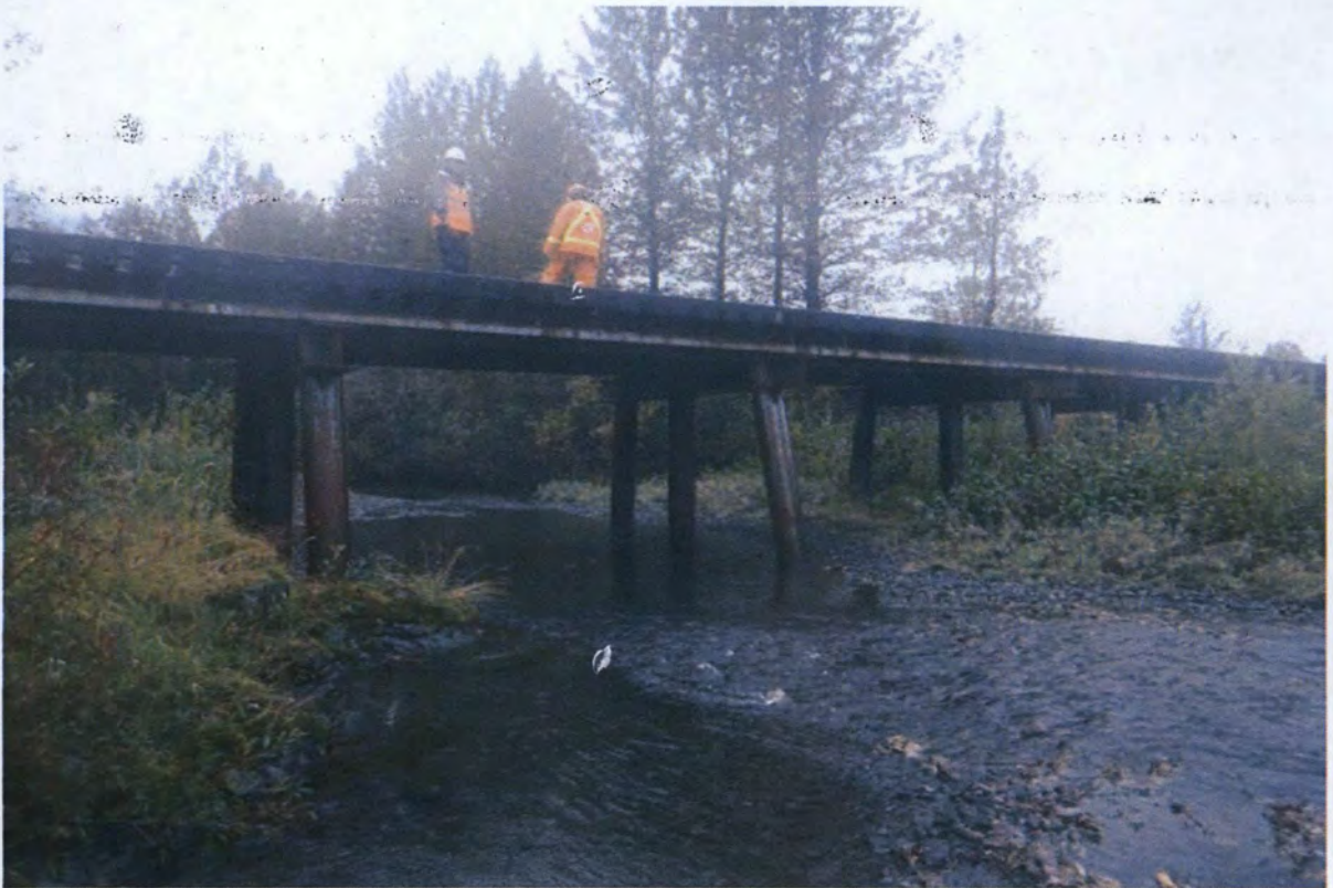
Figure 9. Clear Skookum Creek Bridge. Downstream view.
