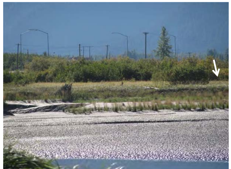
DP-10 Area (From North Side of Twentymile River) September 13, 2010.
