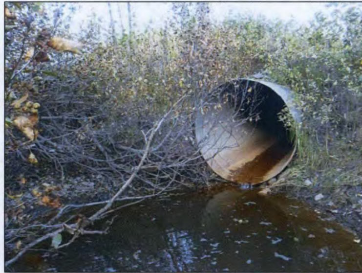
Inset 4. Perched culvert on unnamed tributary to Placer River. September 6, 2016.
