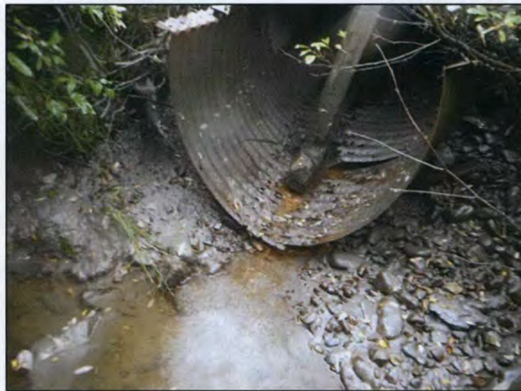
Inset 6. Culvert on unnamed tributary to Placer River. September 6, 2016.
