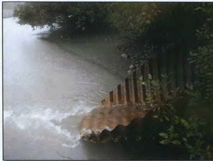
Inset 5. Culvert on unnamed tributary to Placer River. September 6, 2016.
