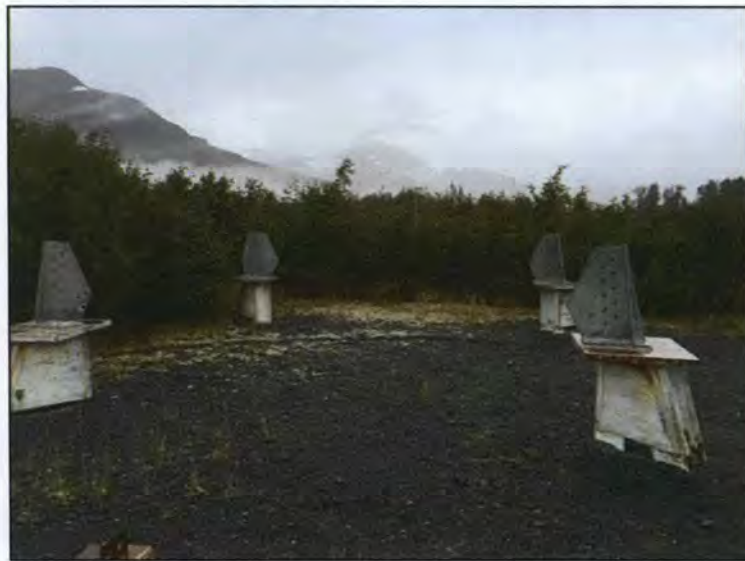
Inset 1. Abandoned microwave tower pad. September 6, 2016.
