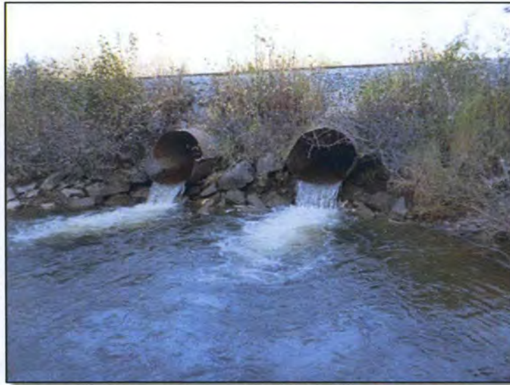
Inset 2. Perched 48-inch culverts on Explorer Creek, outlet view. October 3, 2016.
