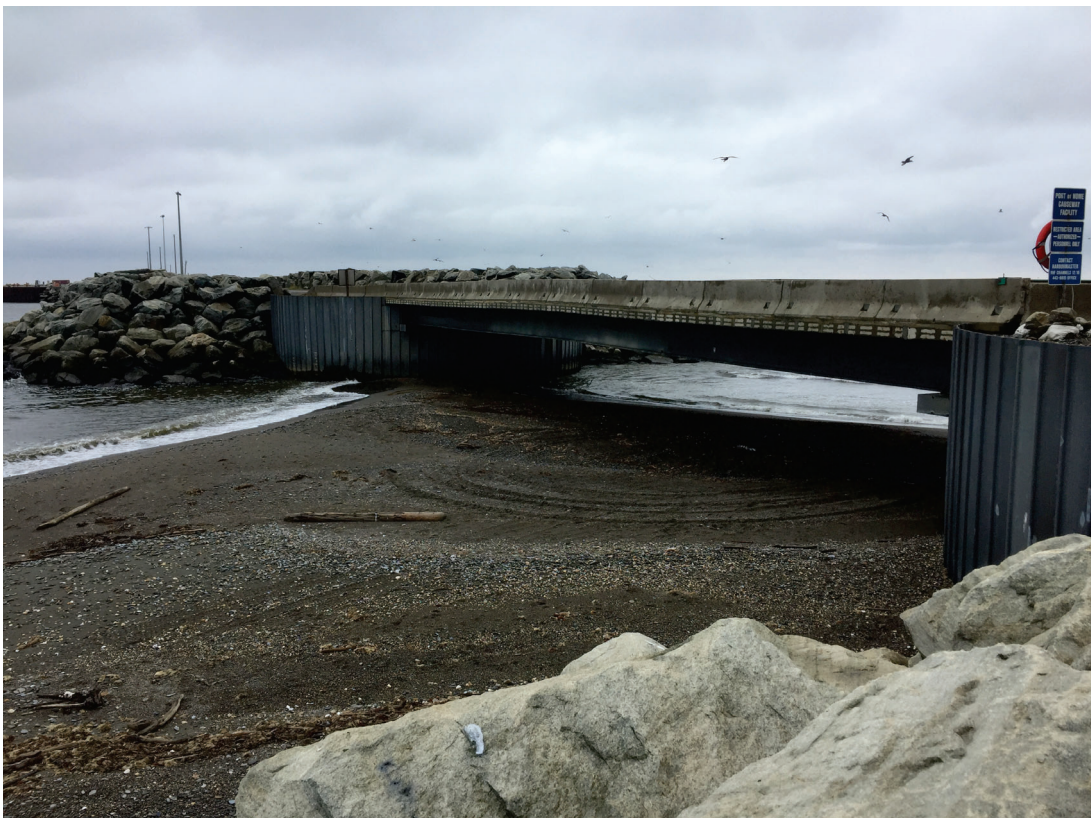
Significant shoaling under the causeway bridge, September 2018
