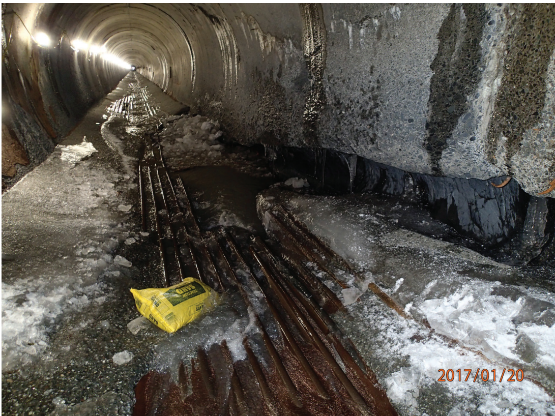
Tunnel damage looking downstream, January 2017
