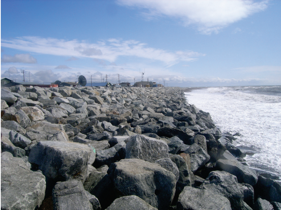
Riprap revetment, July 2011
