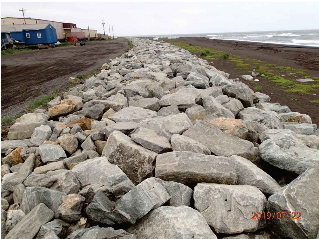
Typical Riprap revetment , July 2019
