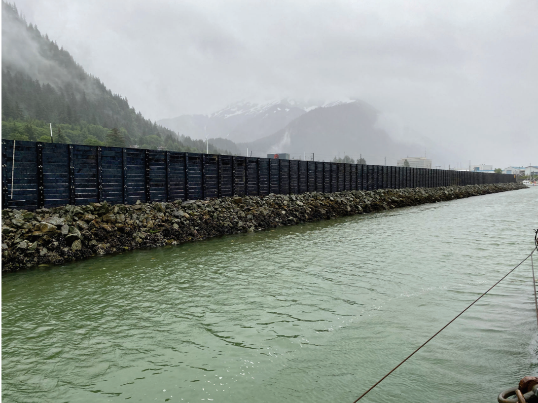
New Wave Barrier at Aurora Harbor, June 2020
