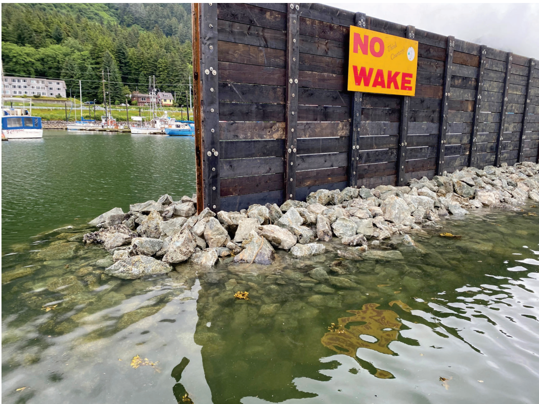
New Wave Barrier at Aurora Harbor, June 2020
