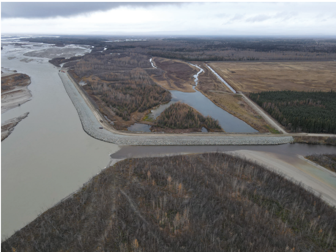
Tanana Sill Groin with completed repairs, September 2022
