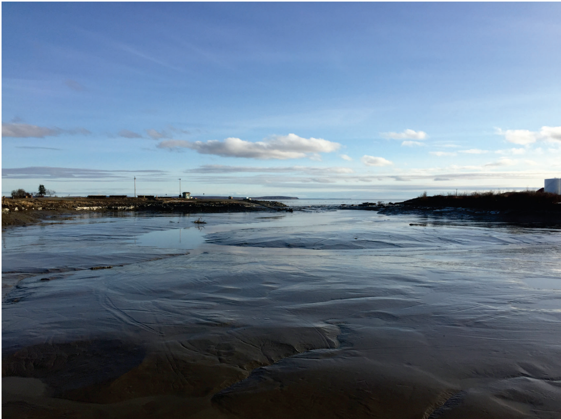
Shoaling in harbor basin prior to dredging, April 2019
