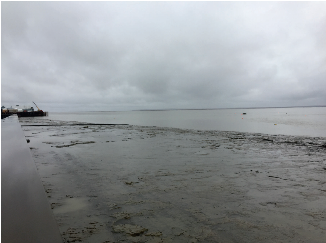
Dredge pipeline route to in-water placement site, May 2016
