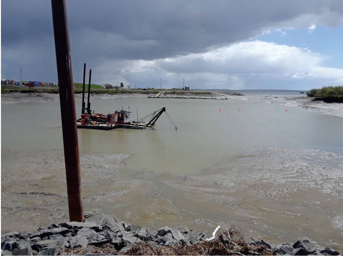
Maintenance dredging of harbor basin, June 2018
