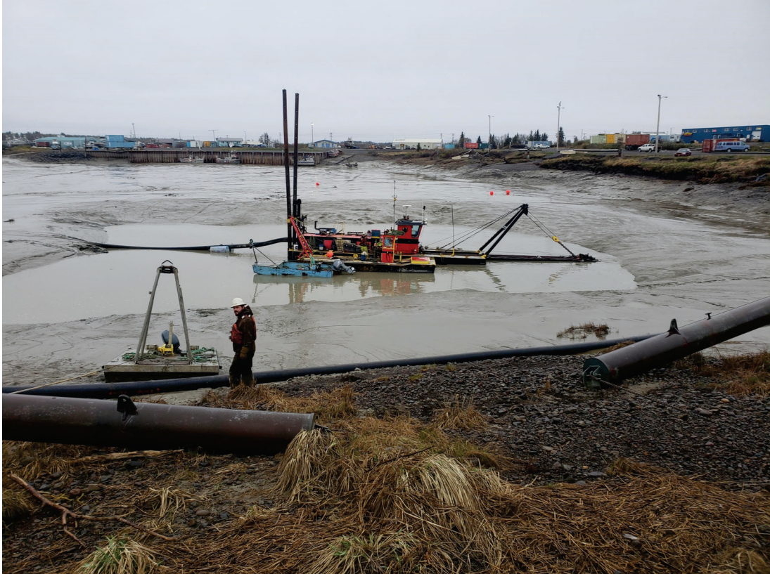
Dillingham Harbor maintenance dredging , May 2020
