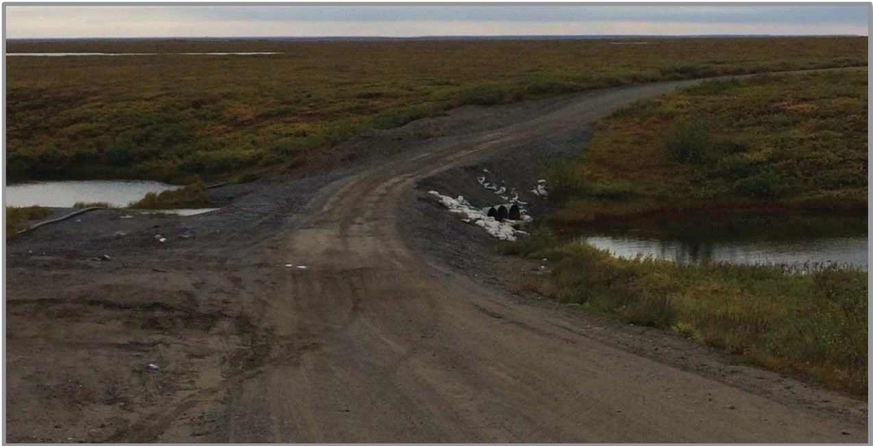
Figure 6: Site 3 Crossing Looking South
