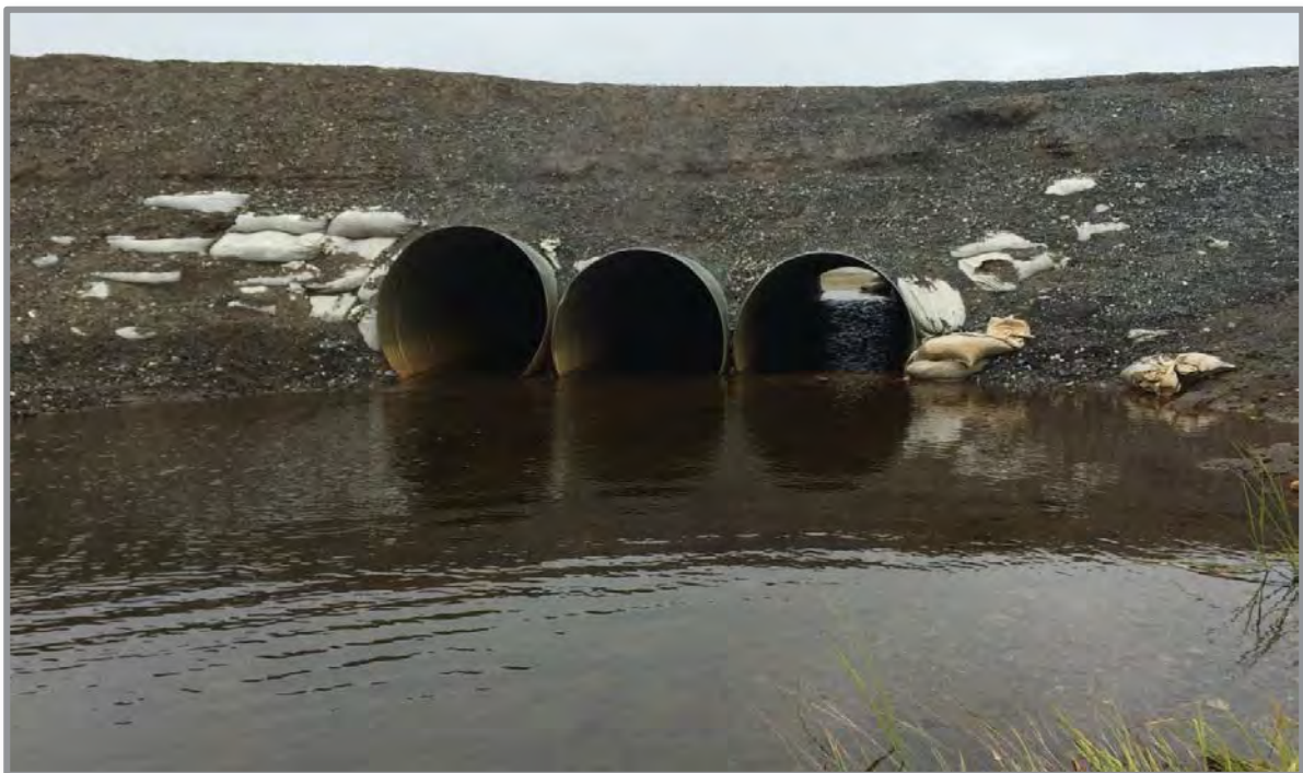
Figure 7: Site 3 Culverts - Downstream Face
