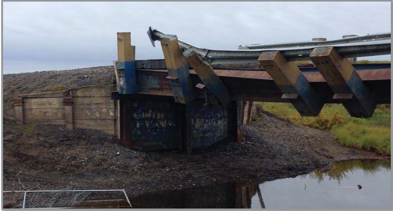
Figure 5: Bridge Abutments at Site 2
