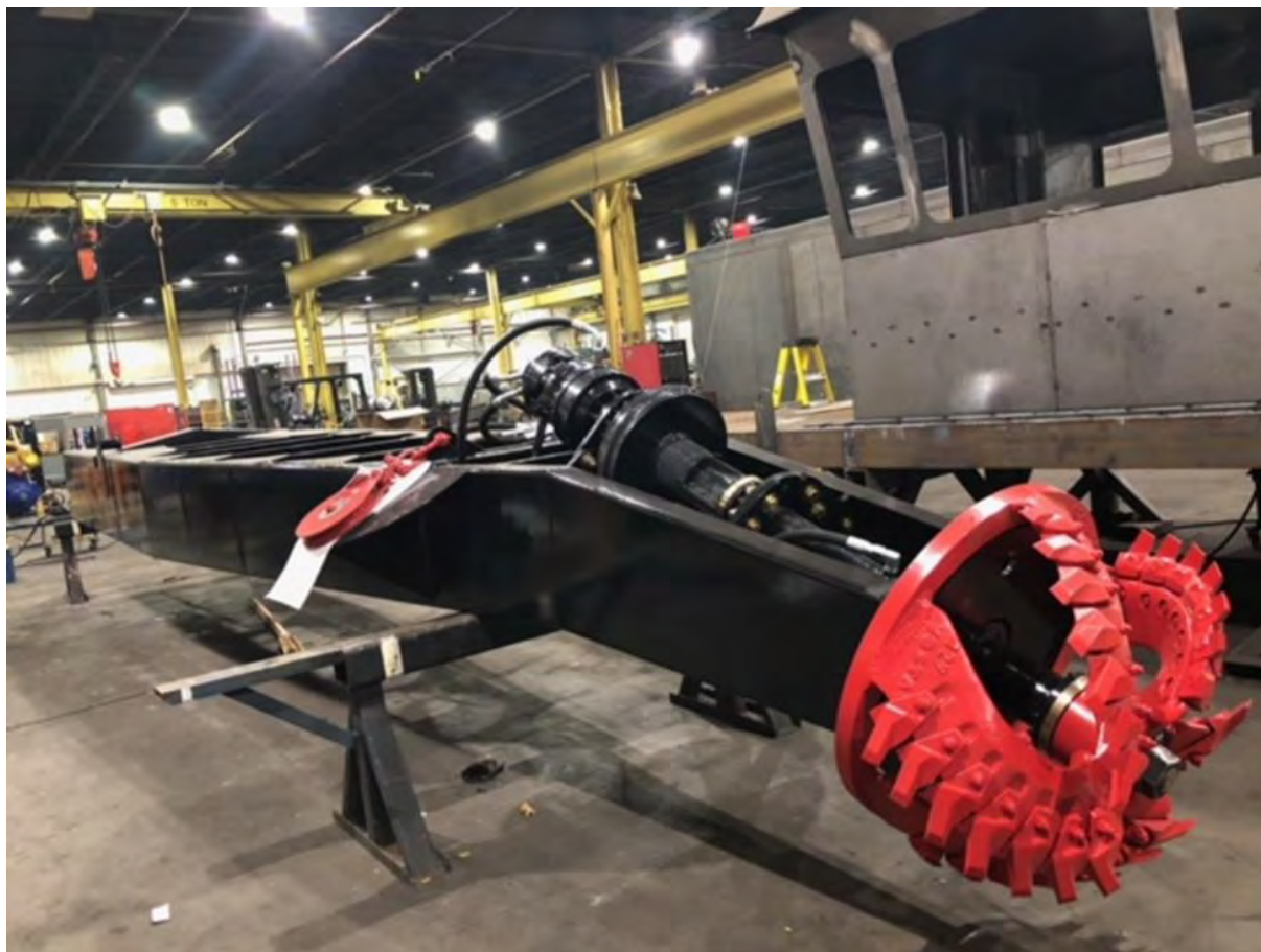
Figure 5-7. Cutterhead and ladder under construction
