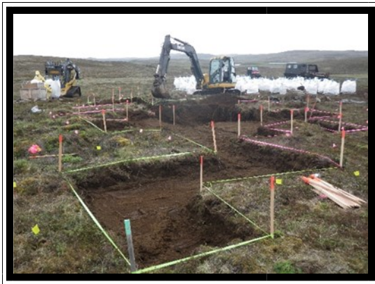
Photograph 3: Excavating PCB-contaminated soil at DS01, 2014 RI
