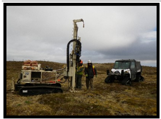
Photograph 4: Drilling at the DS, 2014 RI
