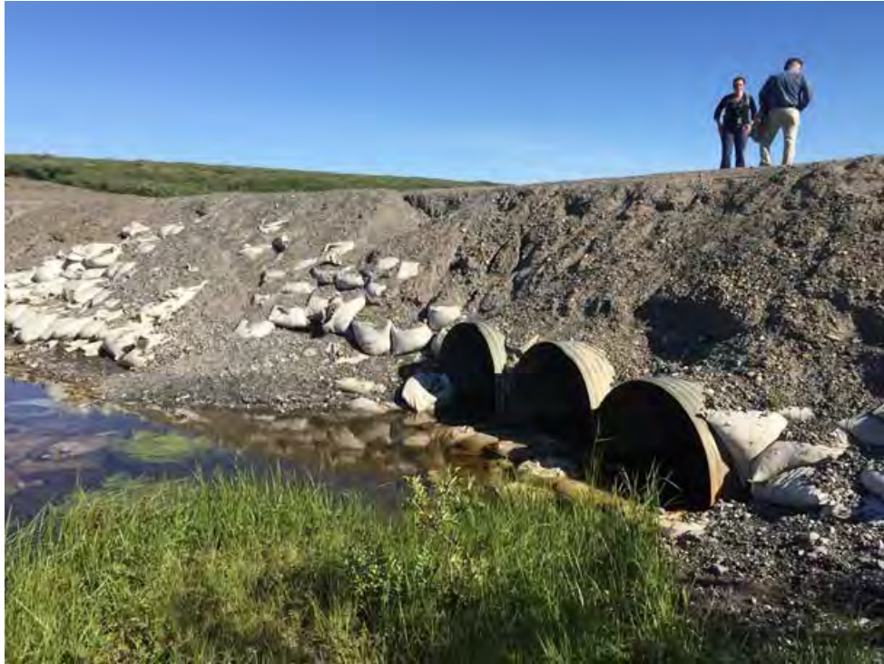
Photo 5. View of upstream side of culverts and sand bag armoring in creek and road embankment.
