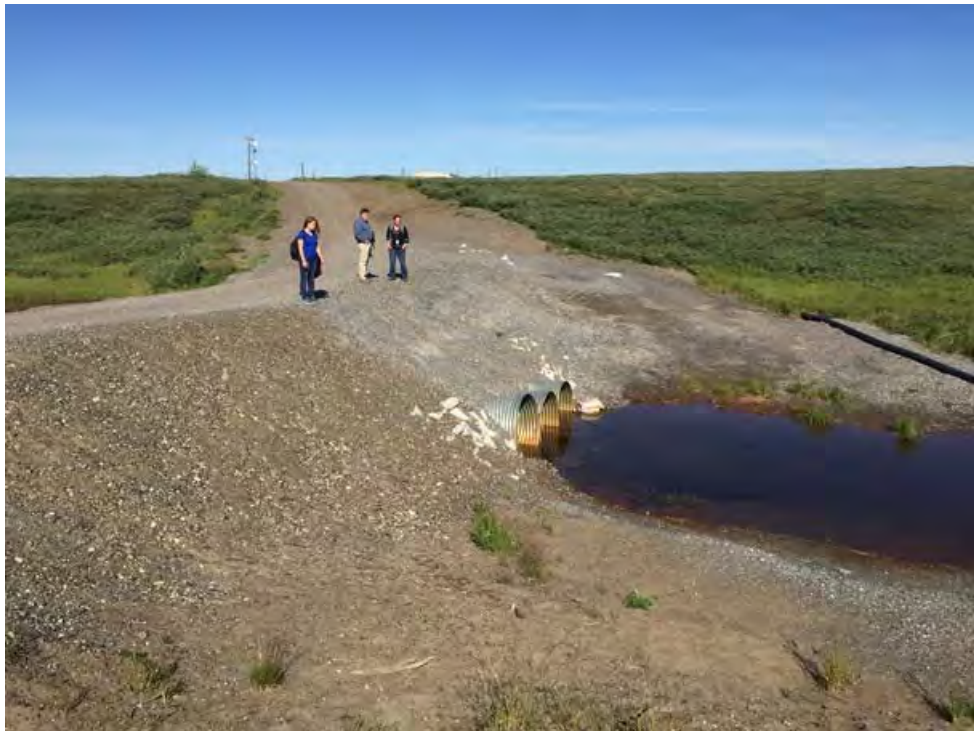
Photo 4. Looking north at downstream side of culverts. The gravel in the stream is from road washouts.
