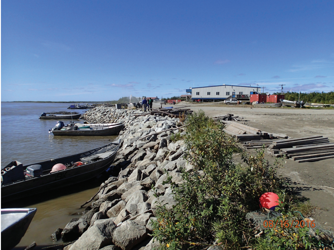
Emmonak revetment downstream of fish processor, August 2016
