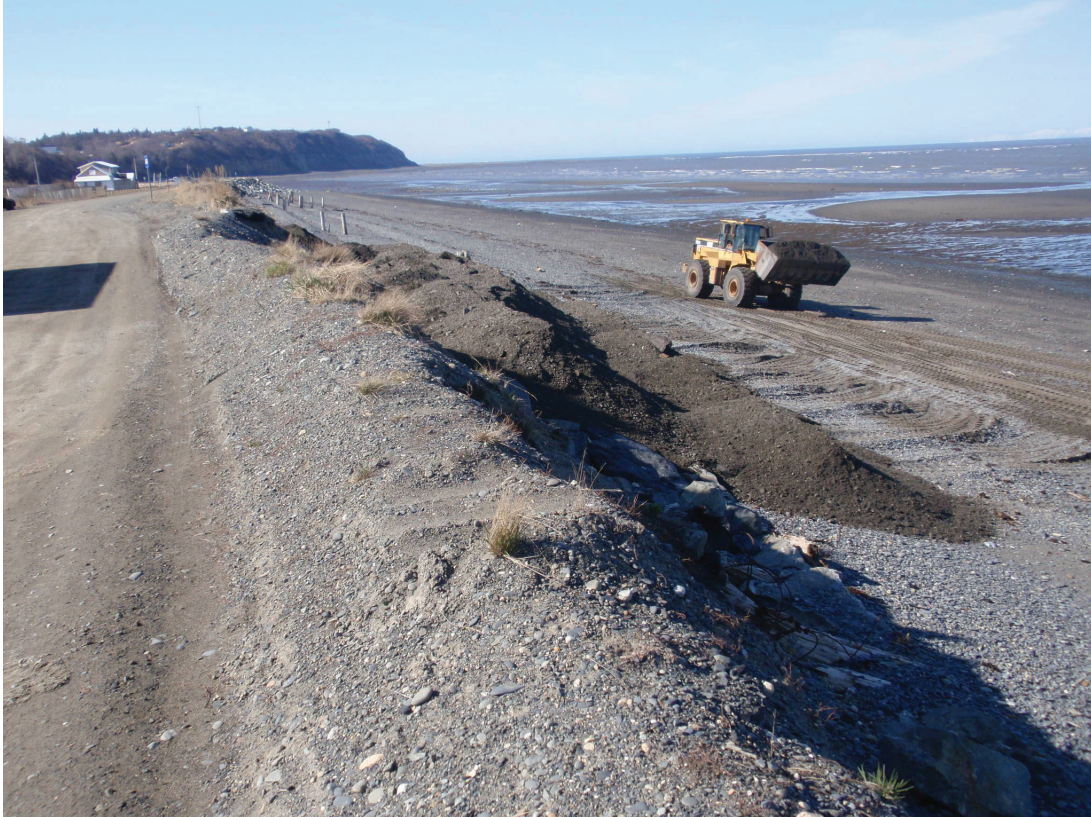
Placement of dredged material on the timber log revetment, May 2019
