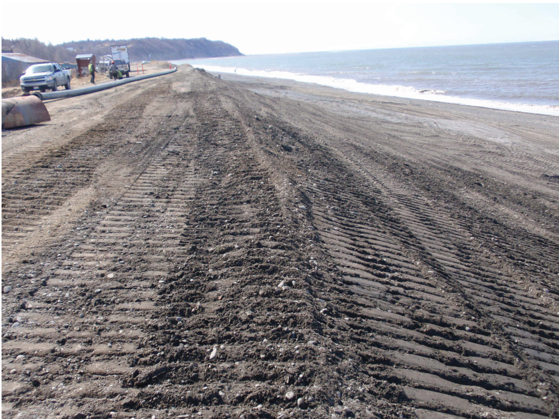
Leveling of dredged material over the revetment, May 2019
