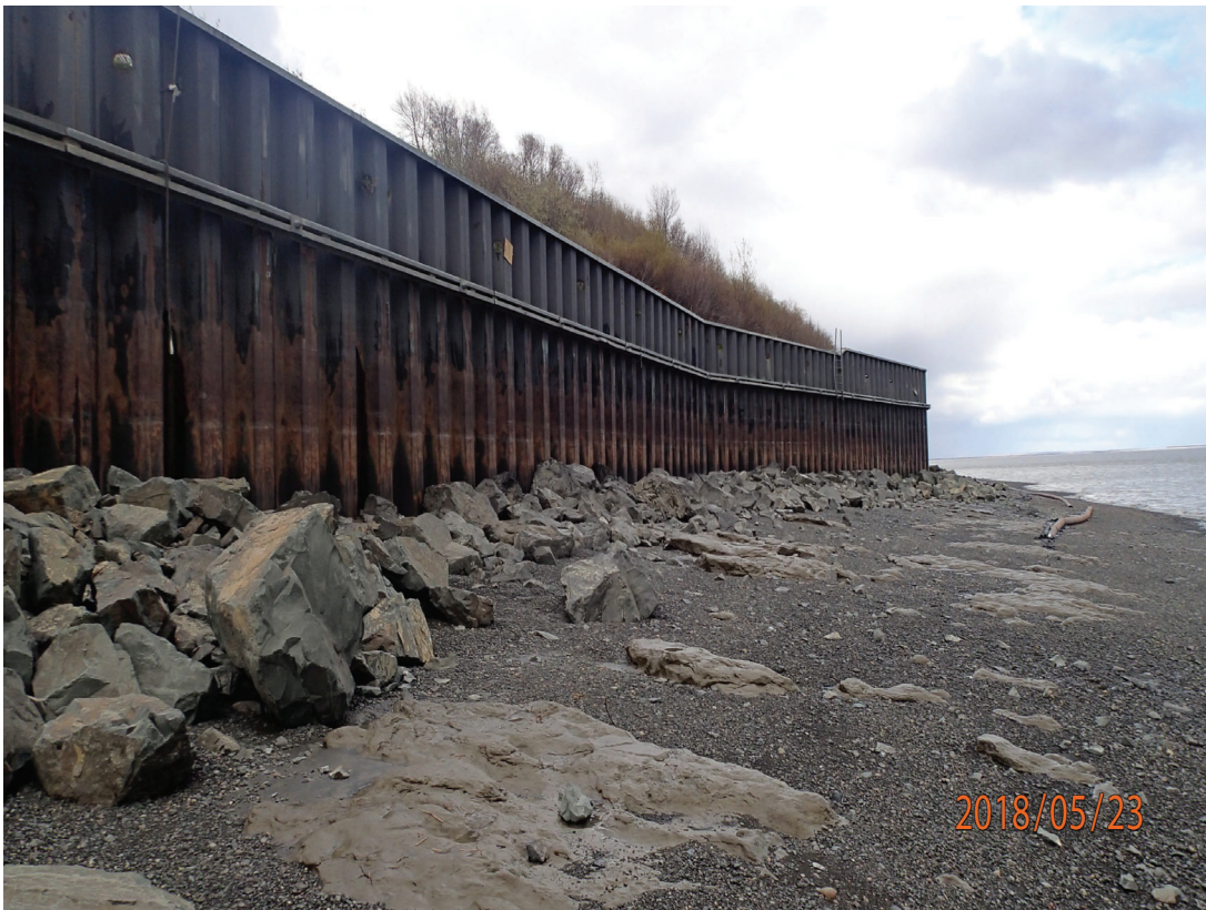
H-pile supported sheetpile bulkhead, May 2018
