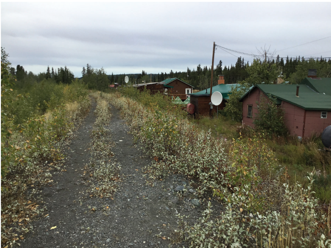
Encroachments within the levee footprint, August 2017
