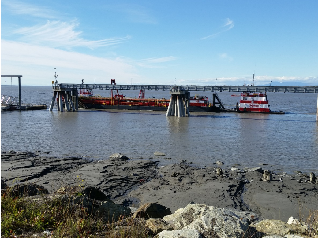
Photo 3: Dredge at work near PA04, looking NW
