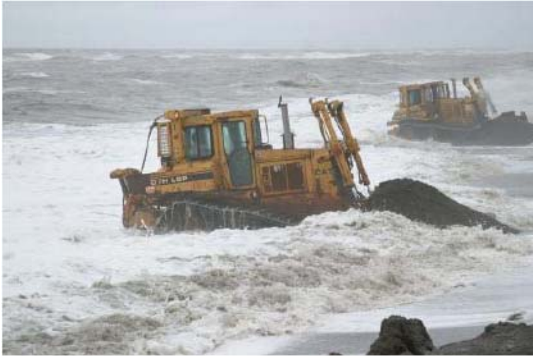
Figure 8: Dozers Rebuilding Beach Berm during Storm
