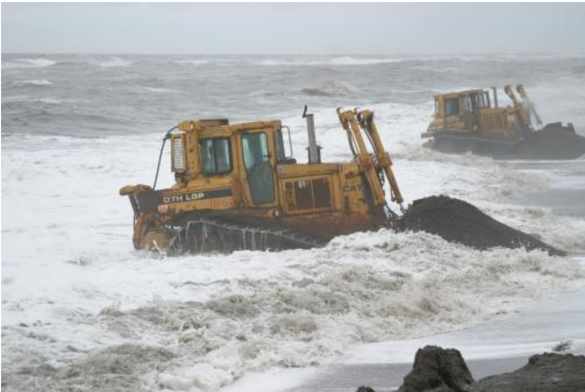
Figure 15. Bulldozer pushing beach material during heavy surf.
