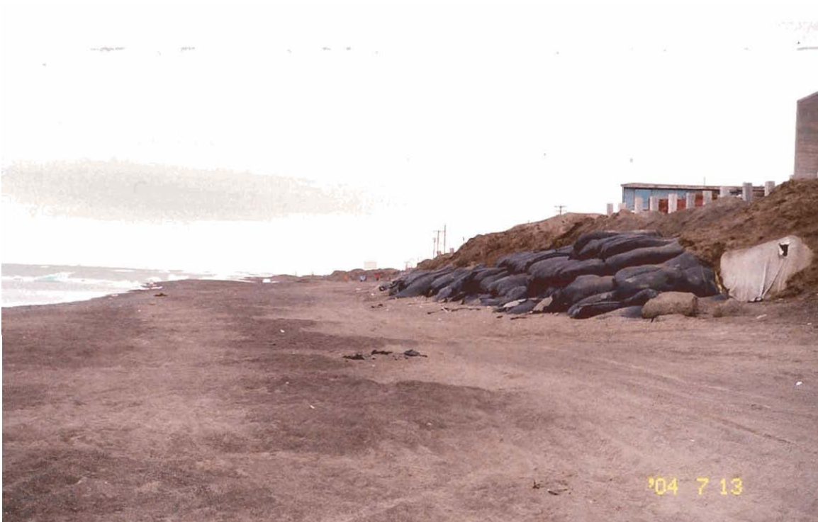
Figure 7. Supersack revetment.
