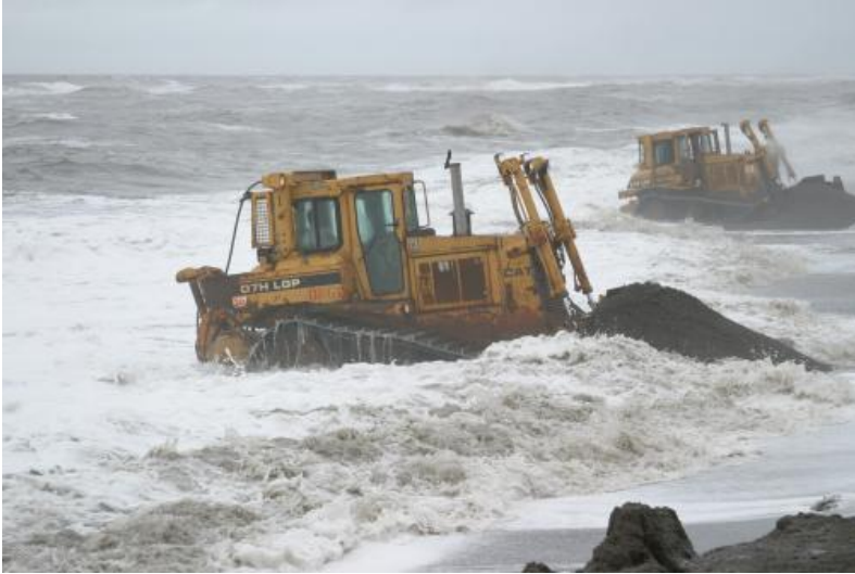
Figure 2. Bulldozer pushing beach material during heavy surf.
