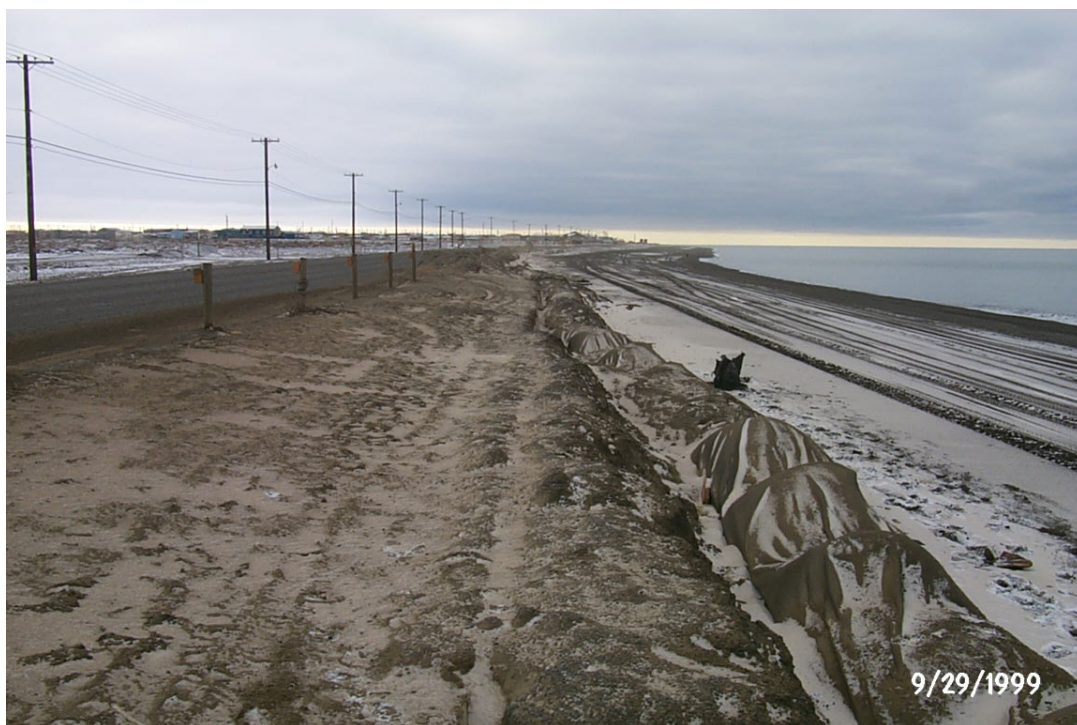
Figure 21. Geotextile tube protection.
