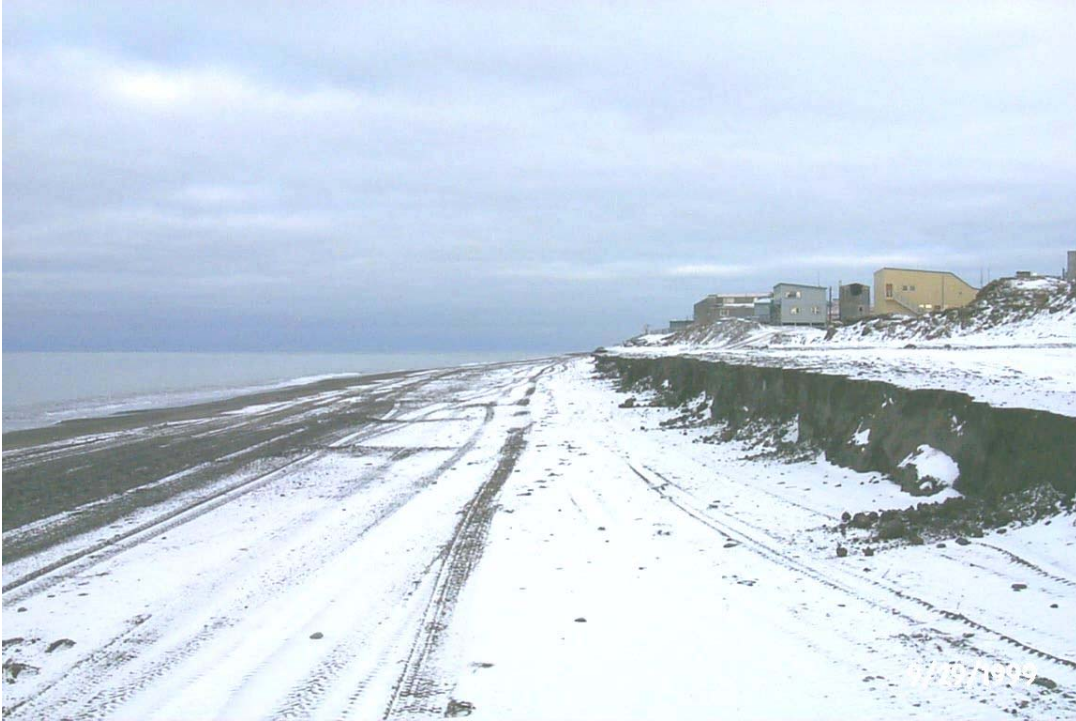
Figure 6. Remains of beach nourishment after storm.
