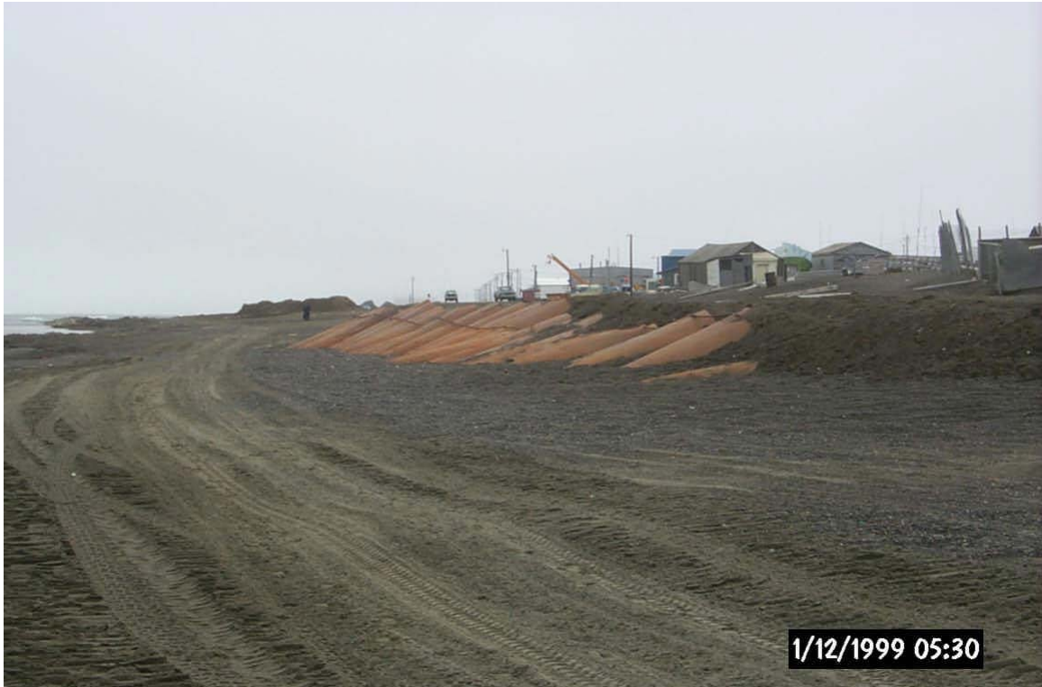
Figure 9. Tar barrels lay on beach at an angle.
