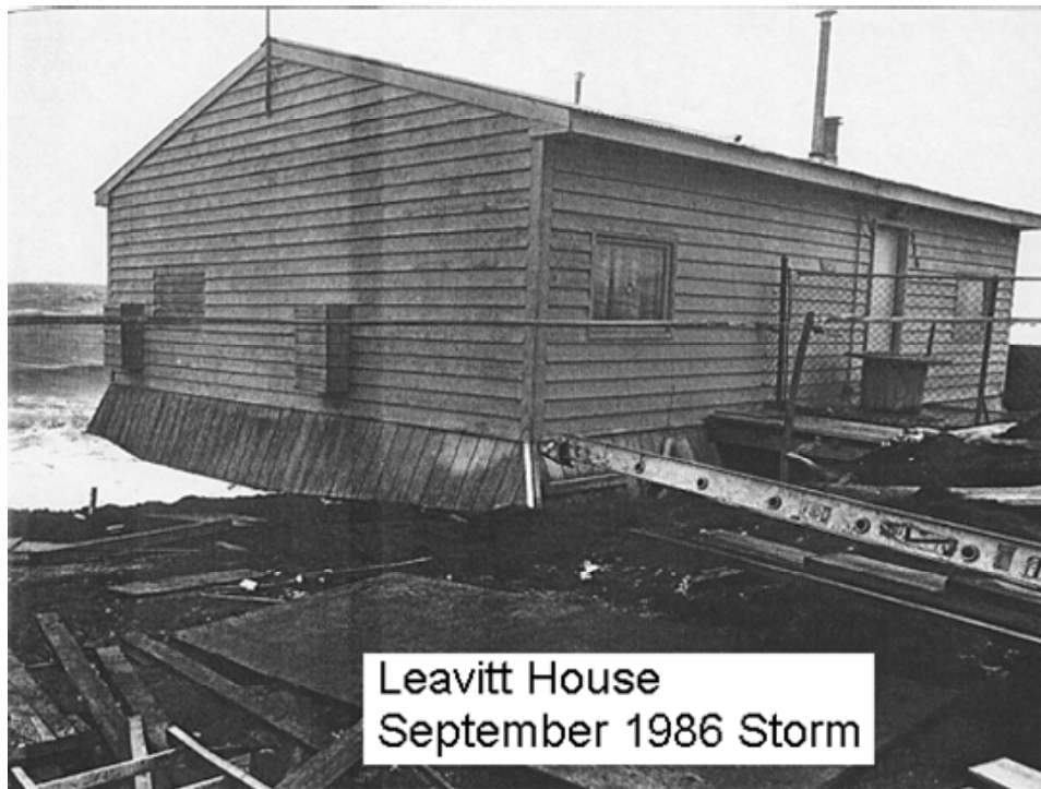
Figure 8. Undermining of structure from erosion.
