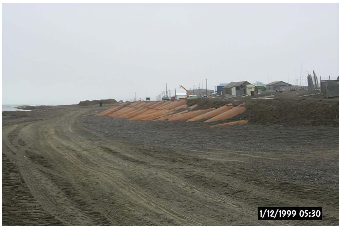
Figure 20. Tar barrels laid on beach at an angle.
