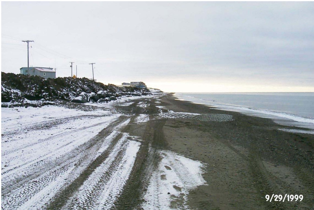
Figure 4. Sacrificial berms placed along road.
