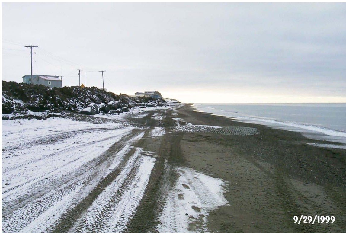
Figure 16. Sacrificial berms placed along road.
