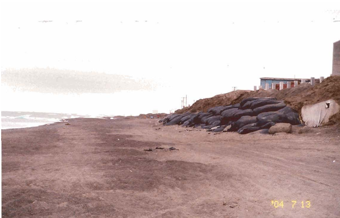
Figure 18. Supersack revetment.
