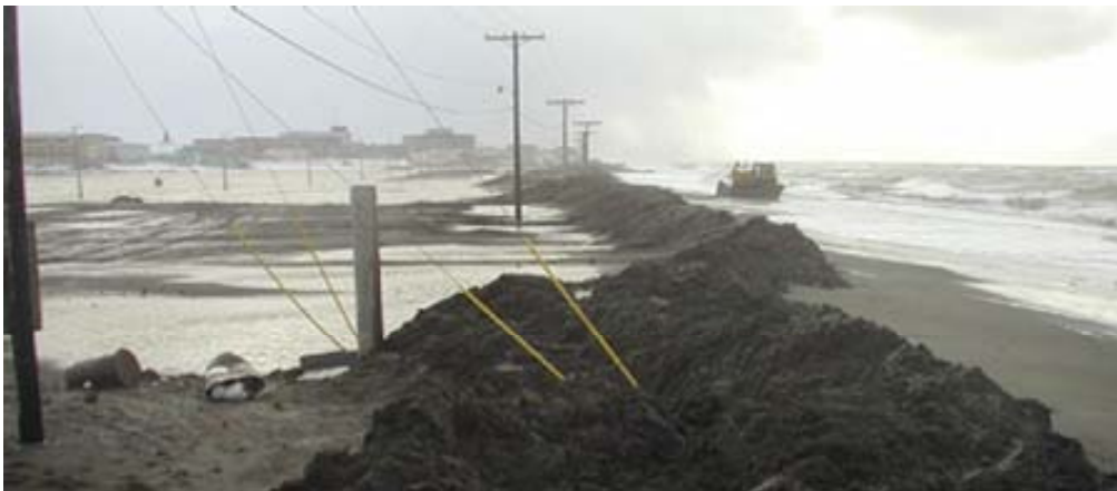
Figure 1. Bulldozer working on the beach building berms at Itasigrook Lagoon
