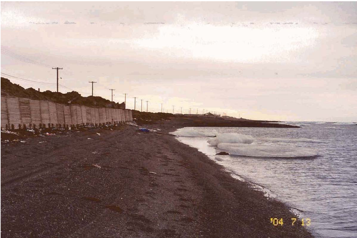
Figure 8. Wooden utilidors backfilled with local material.
