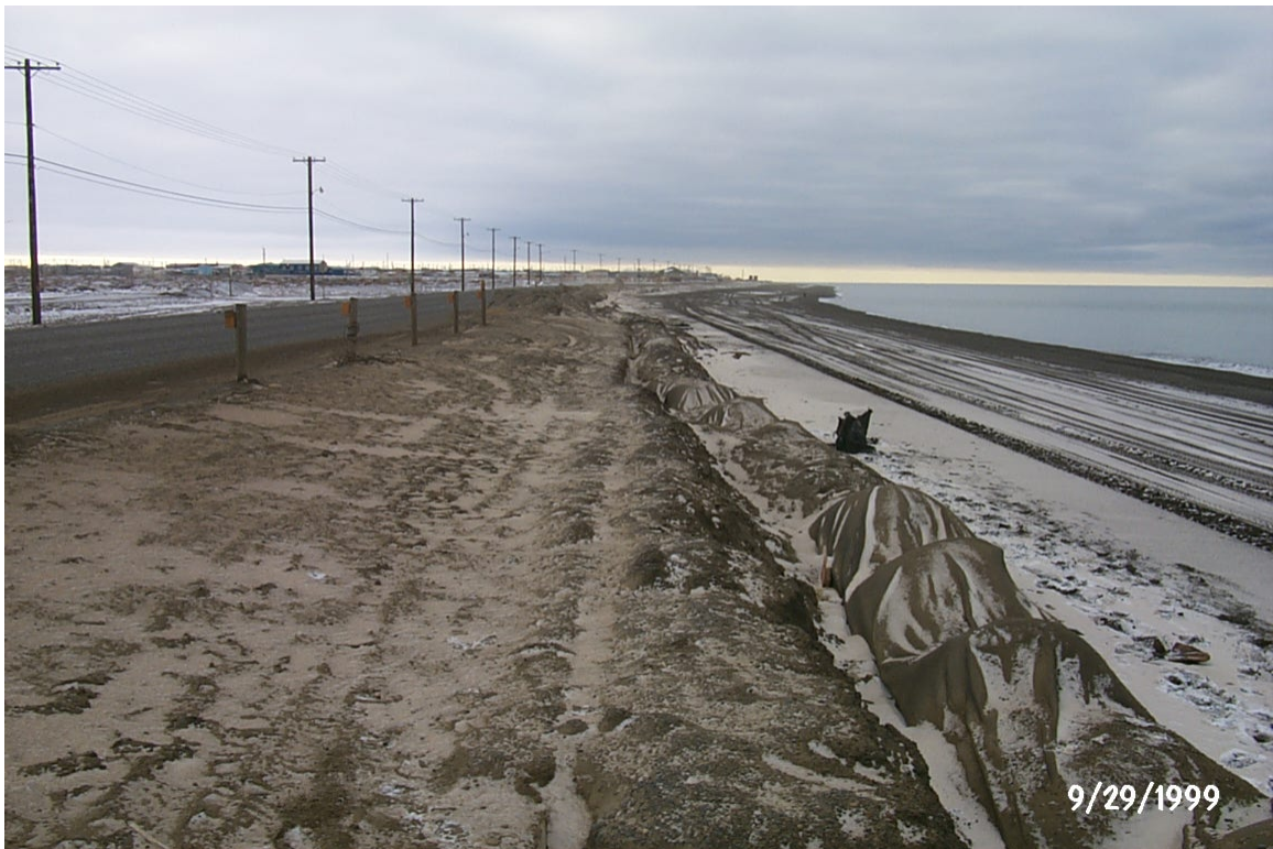
Figure 10. Longard tube type protection.
