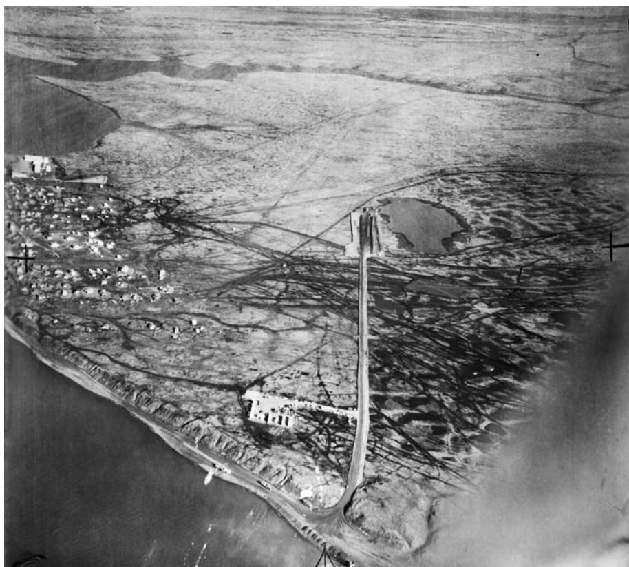
Figure 73. Haul road from the beach leading to the airport during construction.
