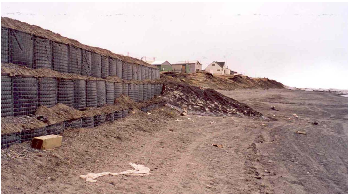
Figure 22. Geotextile fabric encased in a wire basket.
