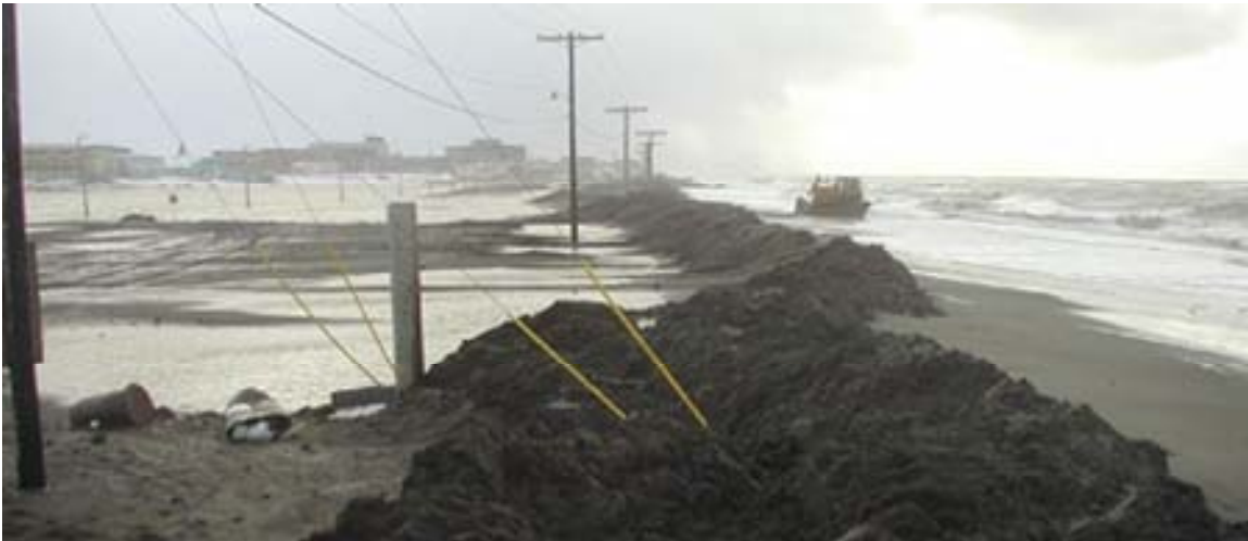
Figure 14. Bulldozer working on the beach building berms.
