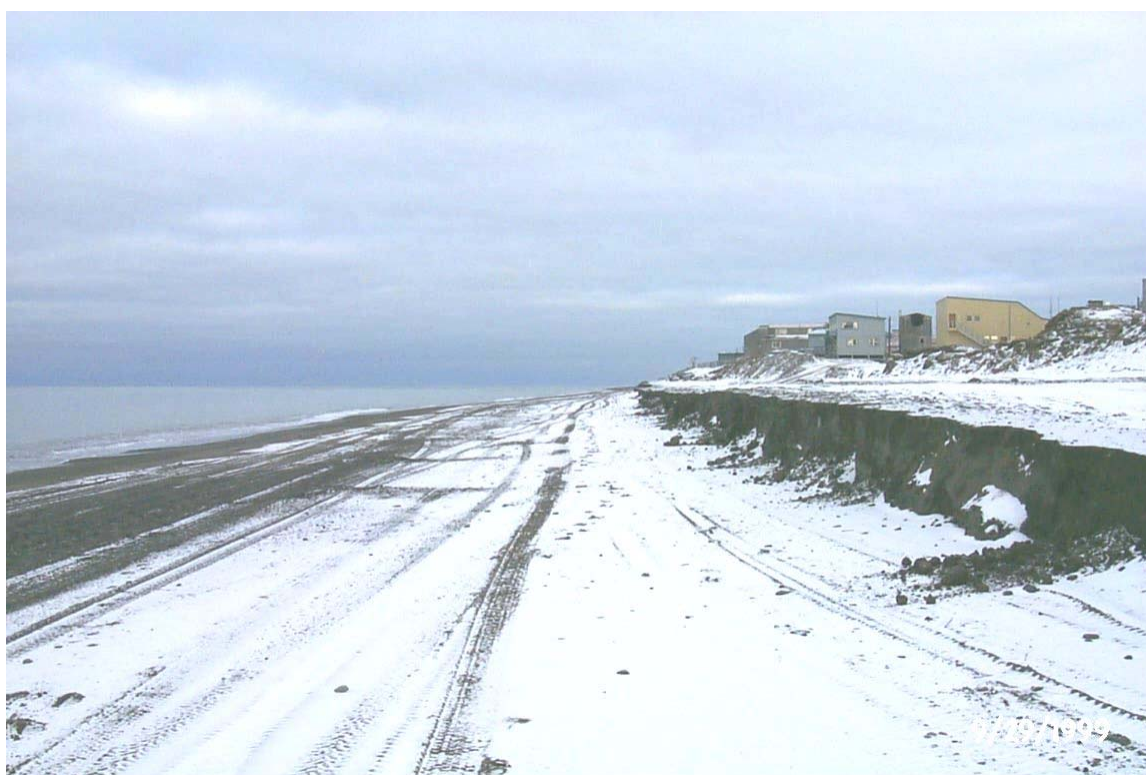
Figure 17. Remains of beach nourishment after storm. The dredging program was never completed. The North Slope Borough's dredge grounded during a storm in 2000.
