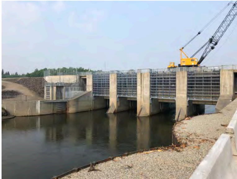
Figure 4. Outlet Control Structure on the Chena River
