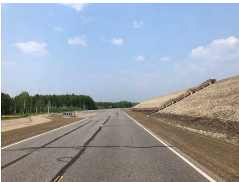
Figure 3. Moose Creek Dam, Laurance Road, and Pedestrian Stair Access
