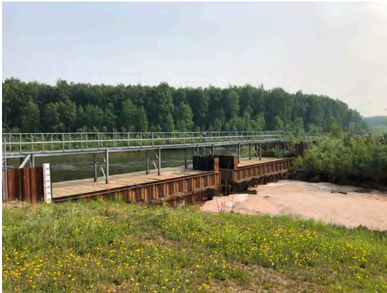
Figure 5. South Seepage Channel Control Gate
