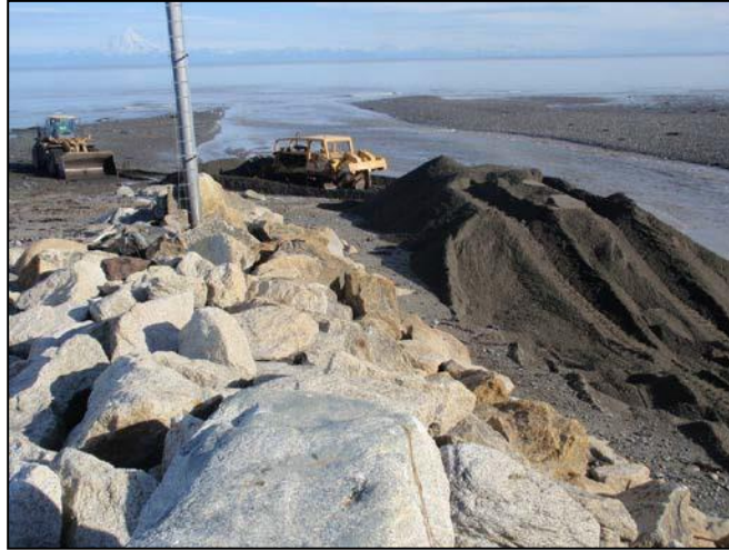
Photograph 1. Construction equipment dredging the Ninilchik SBH entrance channel.
