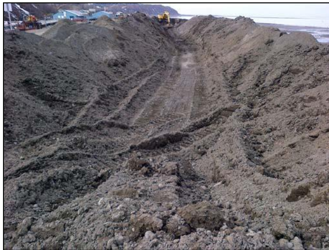
Photograph 2. Constructing the dewatering basin, Ninilchik SBH.
