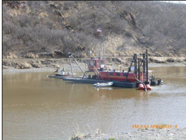
Photograph 3. Hydraulic cutterhead suction pipeline dredge in the Ninilchik SBH mooring basin.
