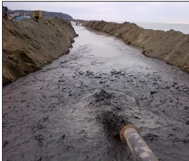
Photograph 4. Dredged material from the mooring basin being discharged into the dewatering basin.
