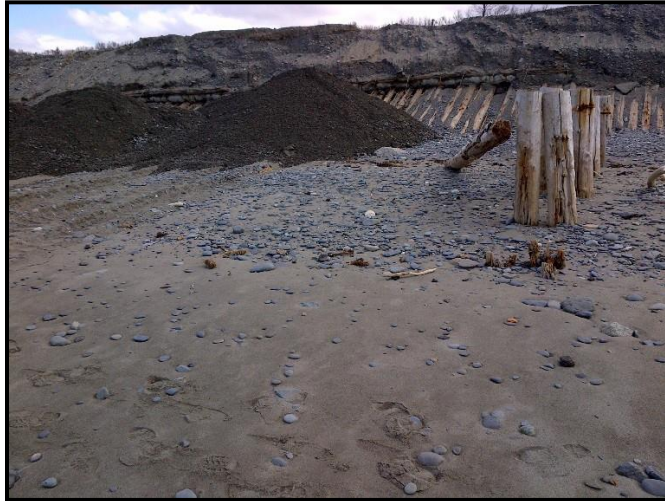
Photograph 5. Dewatered dredged material being placed on damaged and failing shoreline revetment.
