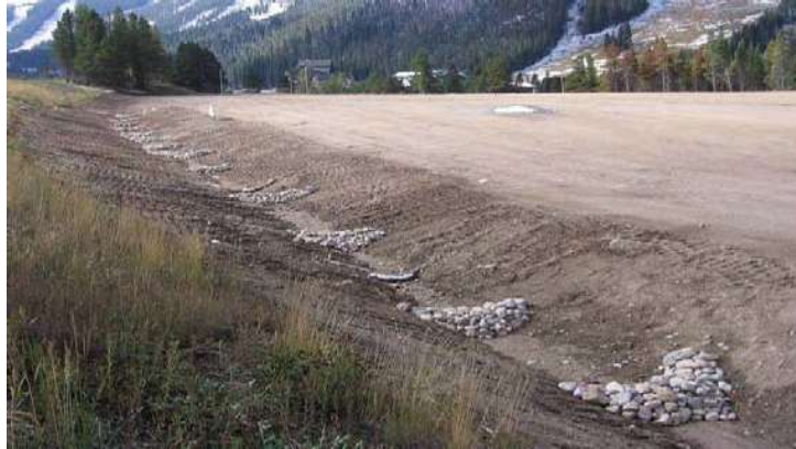
Figure 1: Rock check dams in a roadside ditch. From Mile High Flood District (2024).
