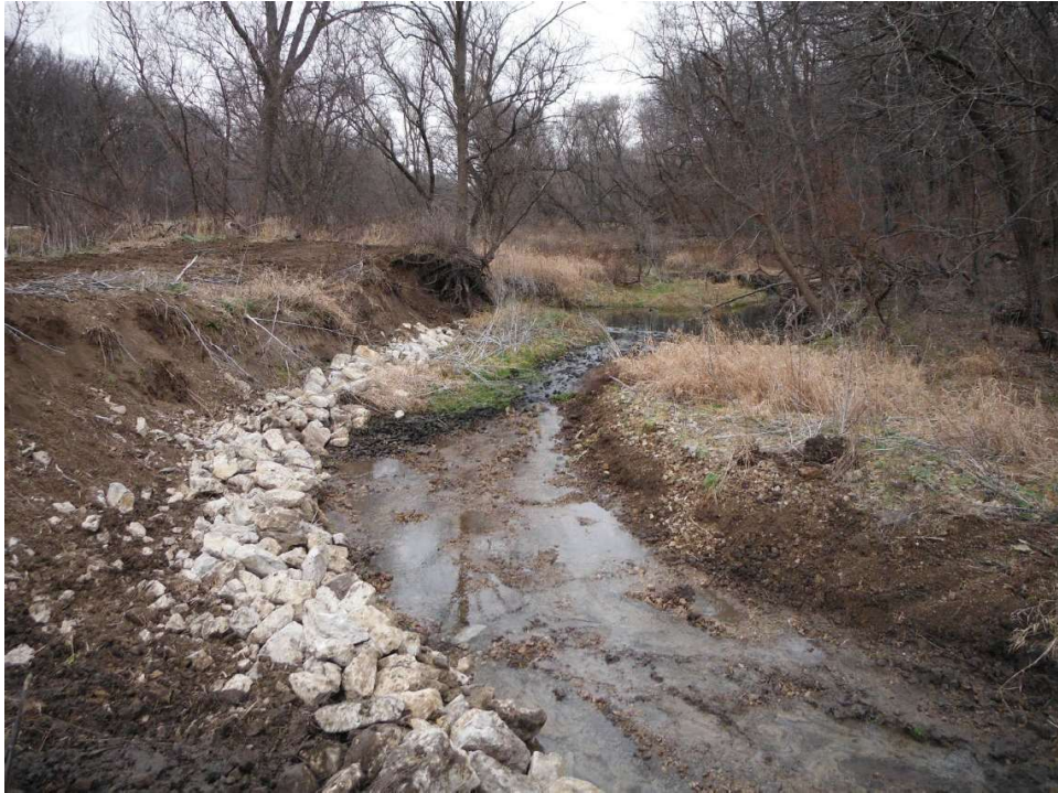
Figure 6: An example of toe slope stabilization. From ERDC's Streambank Erosion and Protection course (2022).
