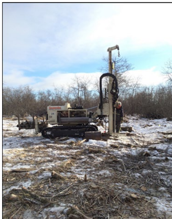
Photo 5: Drilling at the Auto Repair Shop 2007
