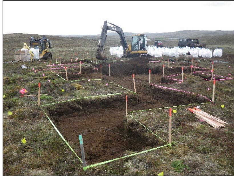
DS01: Excavation of PCB-contaminated soil
