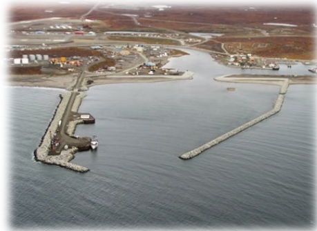
Nome Navigation Improvements IIJA $250M Total Cost: $592M
