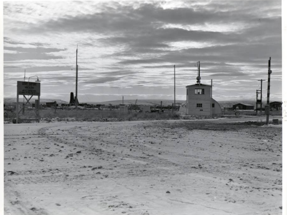
370 - 6 General View of Control Building and surrounding area Umiat.
