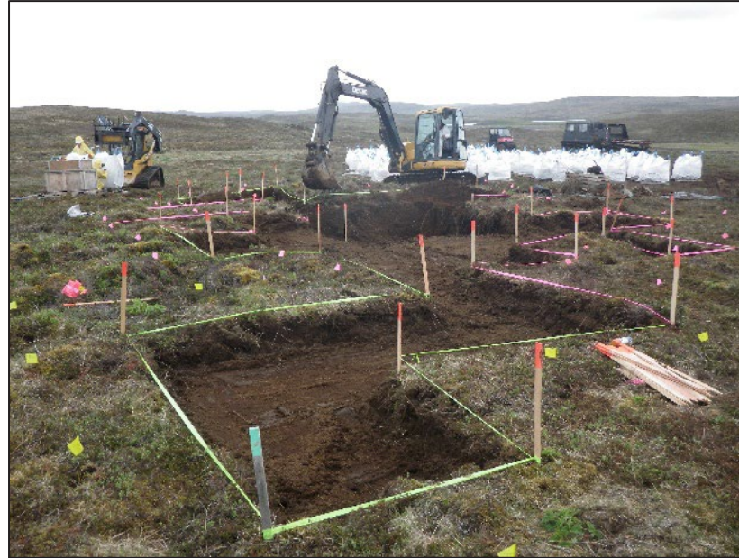
DS01: Excavation of PCB-contaminated soil
