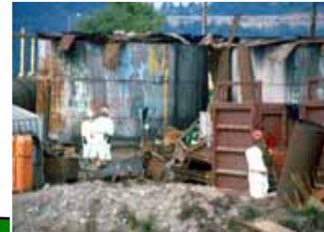
Environmental, Hazardous/Toxic Waste cleanup
