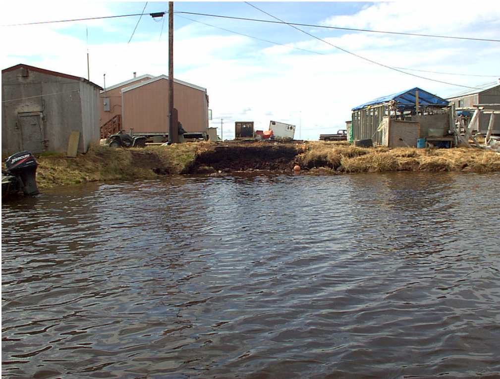
Photo 1: Erosion of the shoreline dated 16 June 2008
