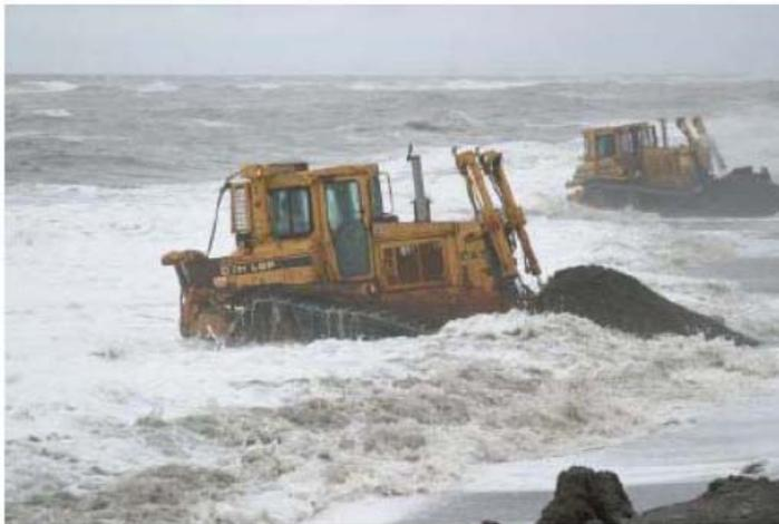
**Photo 3: Rebuilding Beach Berm during Storm. 2000.**
