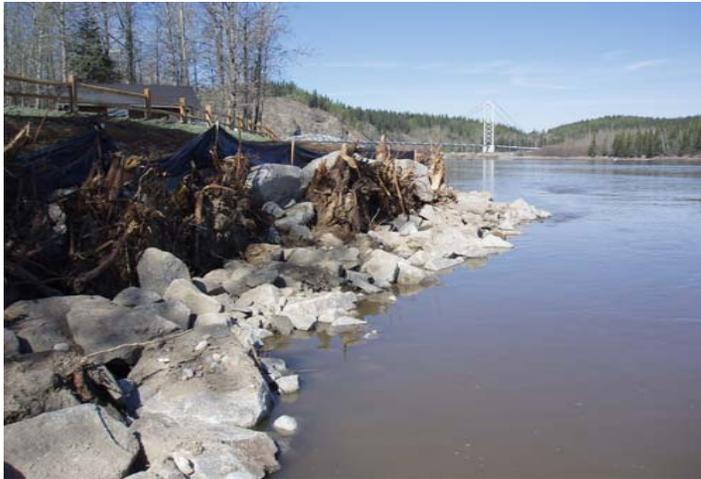
**Photo 1: Toe rock & root wad erosion protection during installation along Tanana River at Rika's Roadhouse. Pipeline crossing is in background, USDA, NRCS photo, 2007.**
